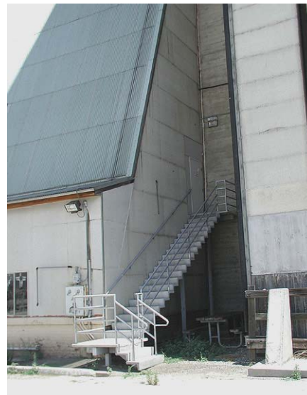
Figure 15. Detail of shed roof connection to parabolic roof, Hangar 2 (Hangar 3 similar).
