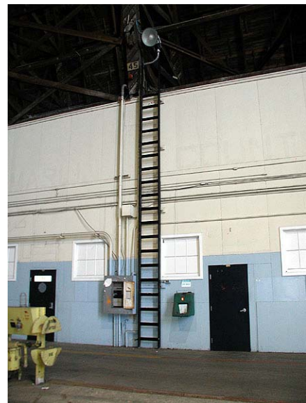
Figure 21. Wood ladder in hangar bay (typical), Hangar 3.
