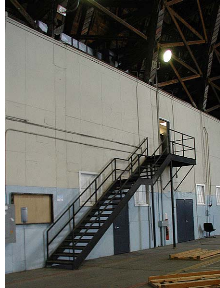
Figure 20. Metal stair (typical), Hangar 3.
