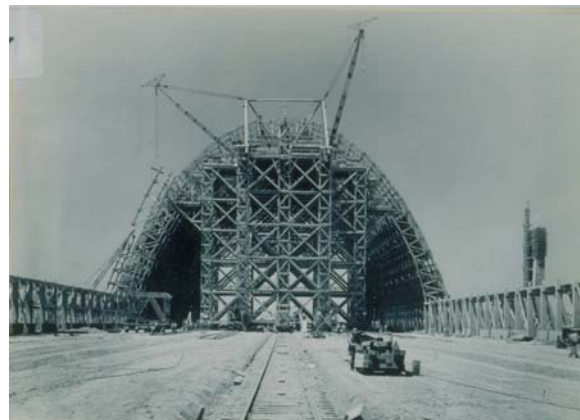
Figure 32. Hangar 3 under construction, June 1943. Source: Moffett Field Historical Museum.
