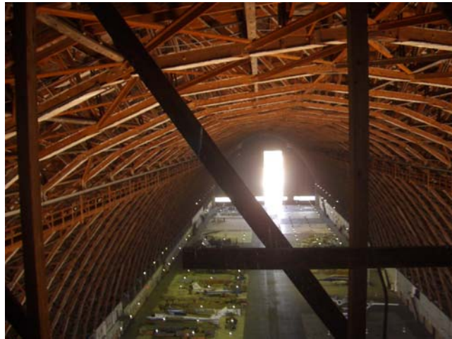
Figure 38. Upper arc of truss assembly, south end, Hangar 2 (Hangar 3 similar).
