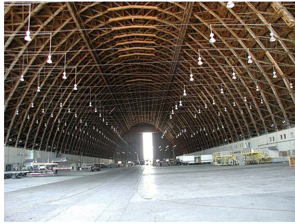
Figure 16. Interior, Hangar 2 (similar to Hangar 3)
