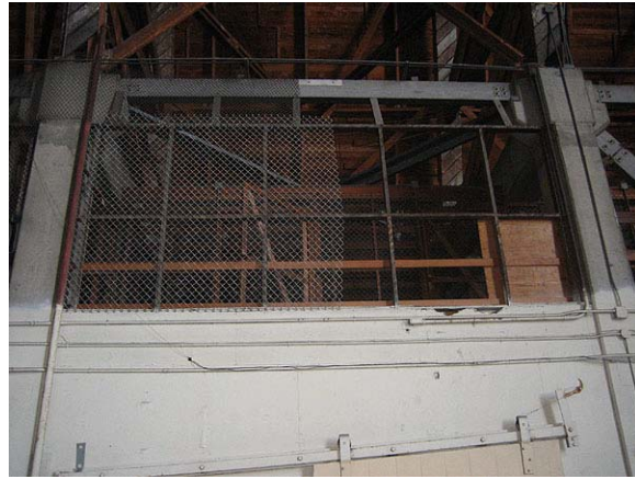
Figure 3a. Upper portion of a concrete bent, interior, Hangar 3.
