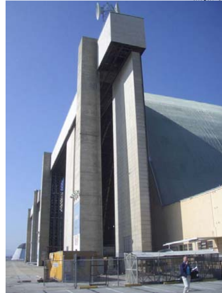
Figure 9. Southeast Corner tower, Hangar 3.
