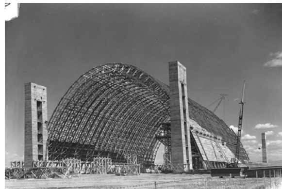
Figure 33. Hangar under construction, 1943. Source: NASA Ames Image Library Server.
