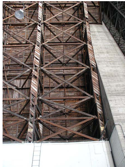
Figure 17. Bents 51 and 50, Hangar 3.
