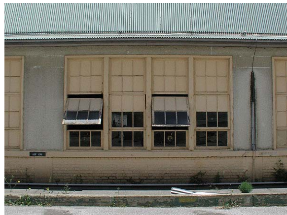
Figure 13. Detail of west lean-to showing brick stem wall, Hangar 3.
