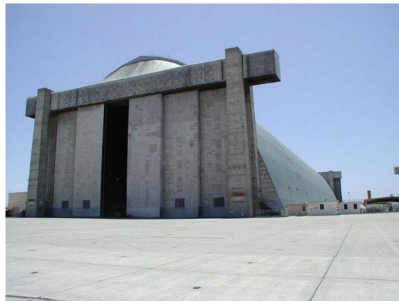
Figure 4. South and east facades, Hangar 3.
