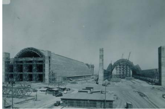
Figure 34. Hangars 2 and 3 under construction, July 1943. Source: Moffett Field Museum.
