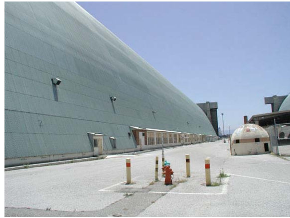
Figure 12. West facade, Hangar 3.
