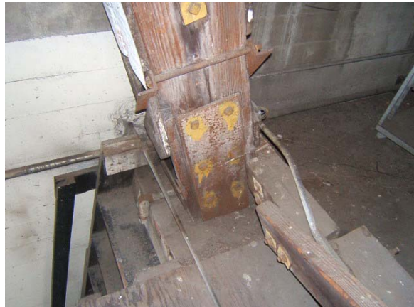
Figure 47: Interface between wood truss and concrete bent, Bent #1, west junction.
