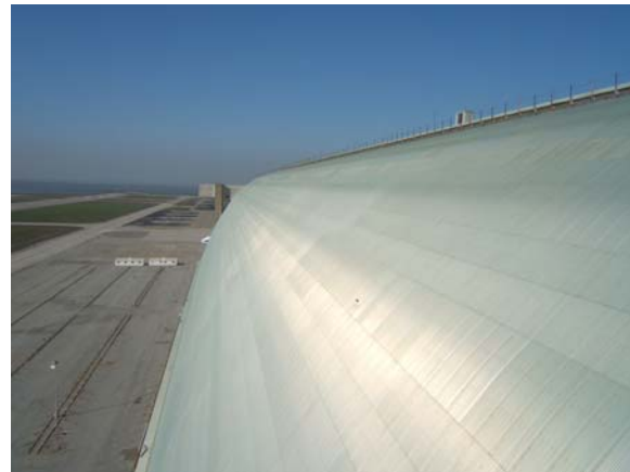
Figure 10. West facing roof, Hangar 3.
