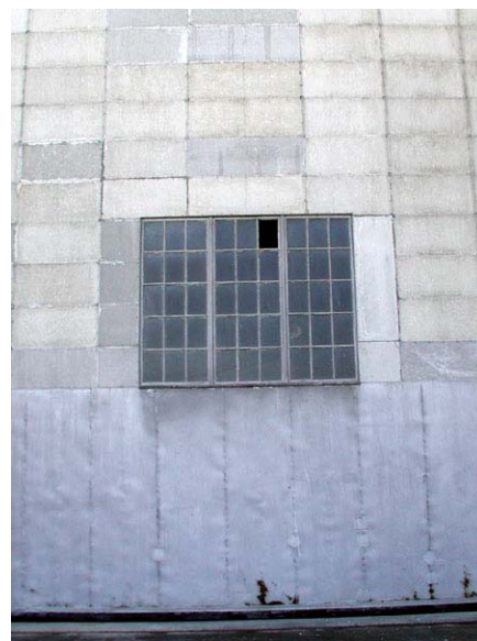
Figure 8. Steel-sash windows on hangar doors, Hangar 3.
