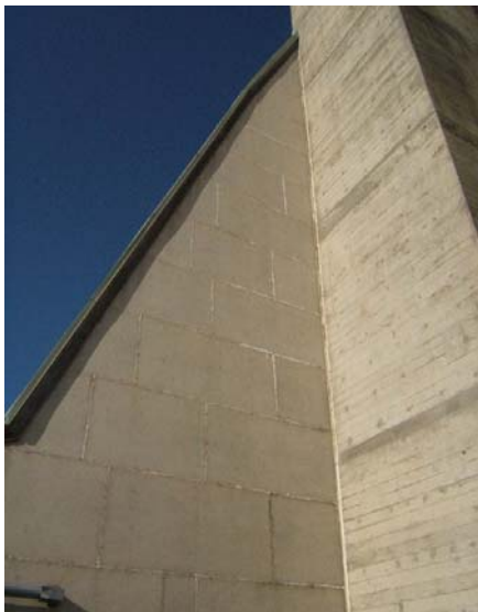
Figure 14. Detail of cement asbestos panels, Hangar 2 (Hangar 3 similar).
