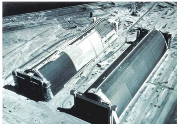
Figure 36. Hangars 2 and 3 near completion, circa 1943. Source: Moffett Field Historical Museum.
