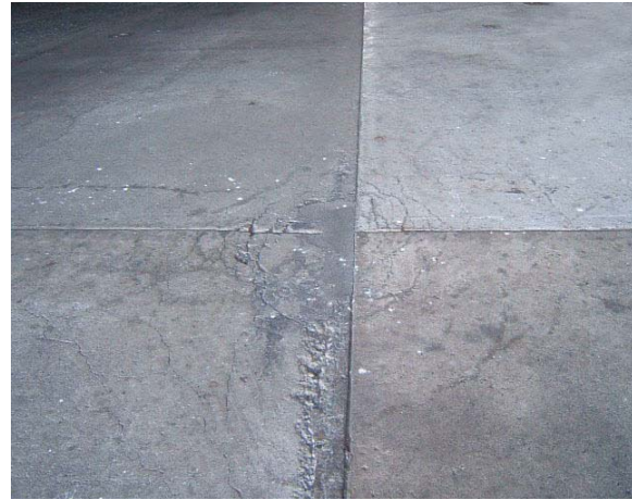
Figure 42 Concrete floor slab (typical), Hangar 2 south entry (Hangar 3 similar).
