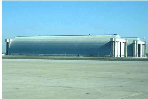
Figure 2. Hangars 2 and 3 (Hangar 3 in background).
