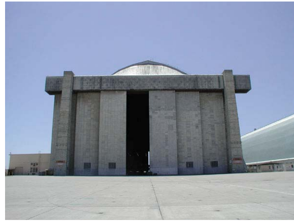
Figure 6. South facade, Hangar 2 (Hangar 3 similar).
