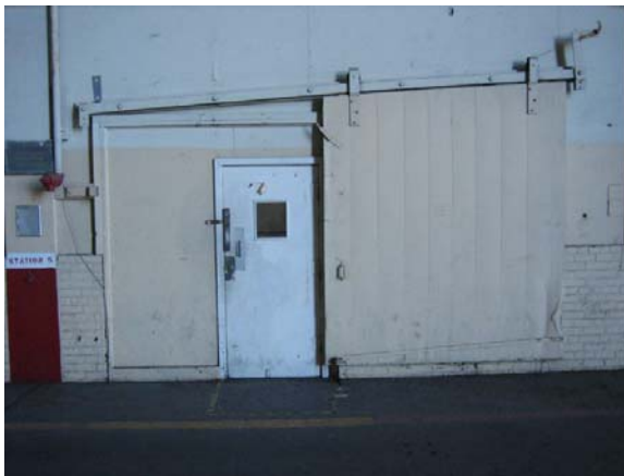
Figure 23. Warehouse door, Hangar 2 (Hangar 3 similar).
