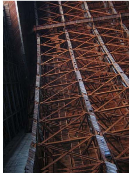
Figure 41 Braces, ladder and catwalk assembly between Bents #1 & #2, Hangar 2 (Hangar 3 similar).
