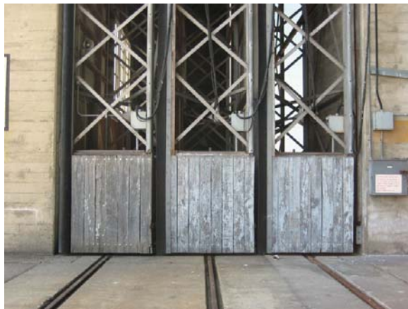
Figure 7. Hangar doors, Hangar 3.
