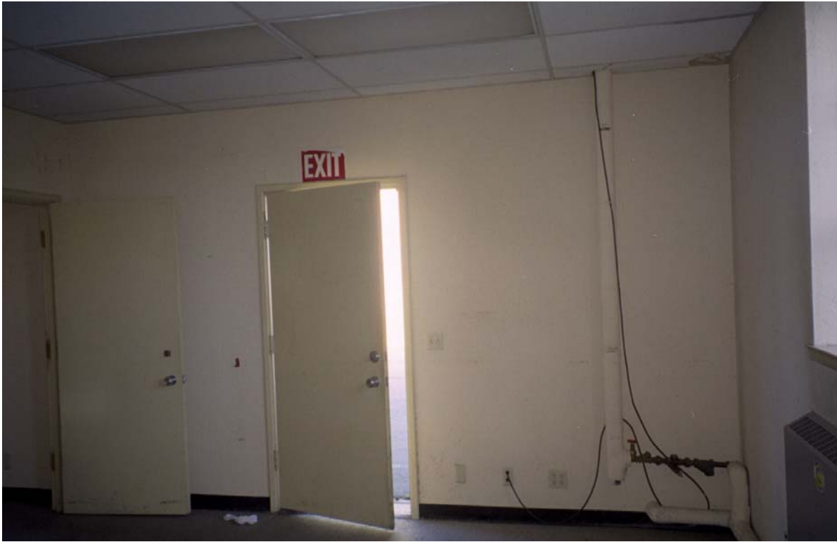
Interior, Building 24 December 13, 2001
