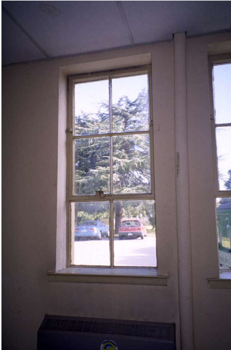
Typical Window, Building 24 December 13, 2001
