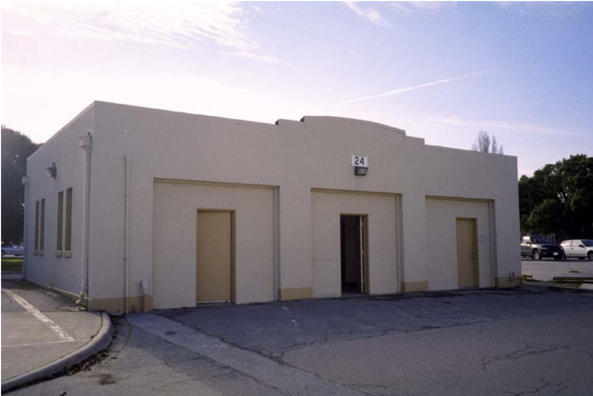
Front Elevation, Building 24 December 13, 2001
