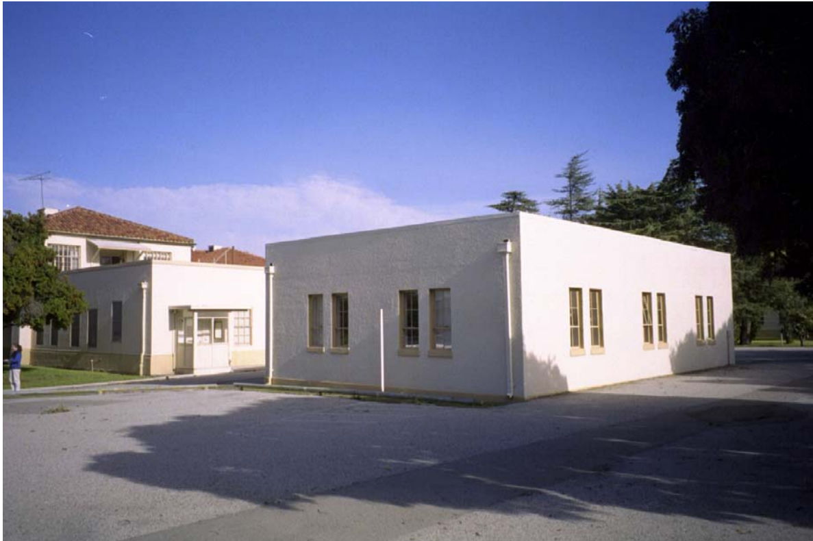
Side and Rear Elevation, Building 24 December 13, 2001
