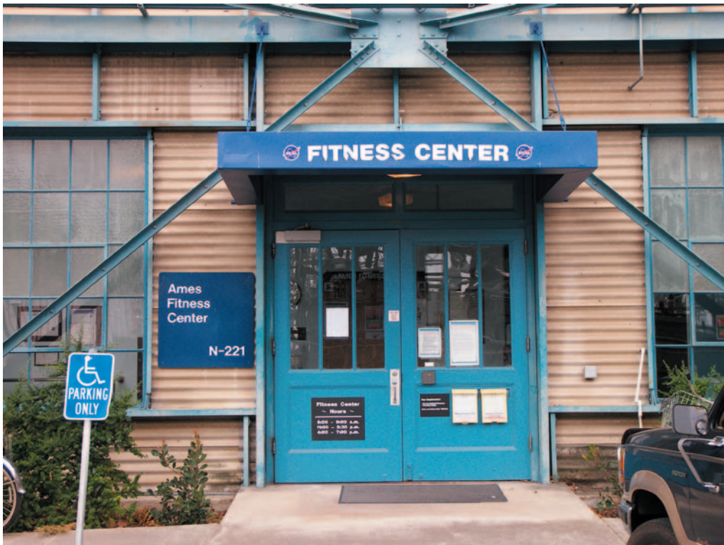
Figure 17. Fitness Center entry
