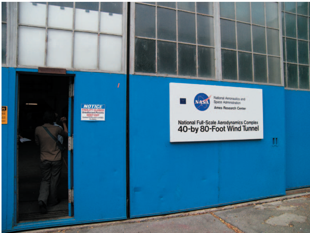
Figure 25. East entry of 40 by 80 Foot Wind Tunnel
