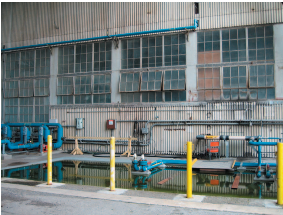
Figure 20. Windows at the courtyard with hopper segments
