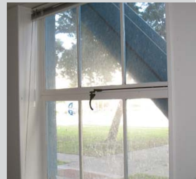
Illustration 5. Multi-lite metal sash windows at ground floor are a significant feature. (Source: ARG, October 2006)
