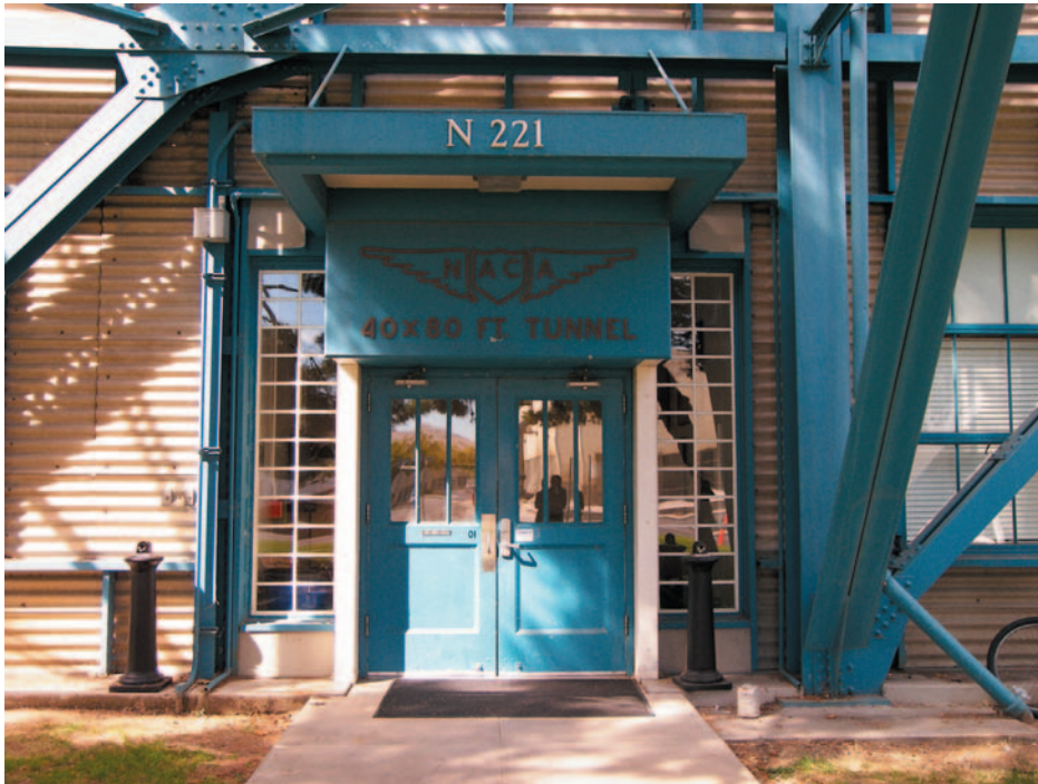
Figure 12. East entry of the 40 by 80 Foot Wind Tunnel with the original name "NACA"
