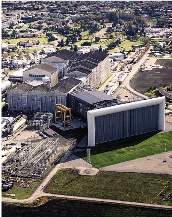
West and North Elevations of Building N-221.
