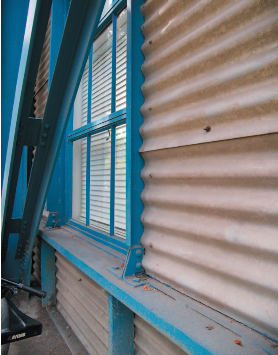
Figure 14. Wall, window, and steel structure
