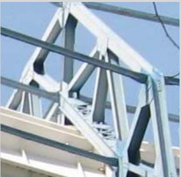
Illustration 2. Geodesic steel bent exoskeleton is a significant feature. (Source: ARG, October 2006)
