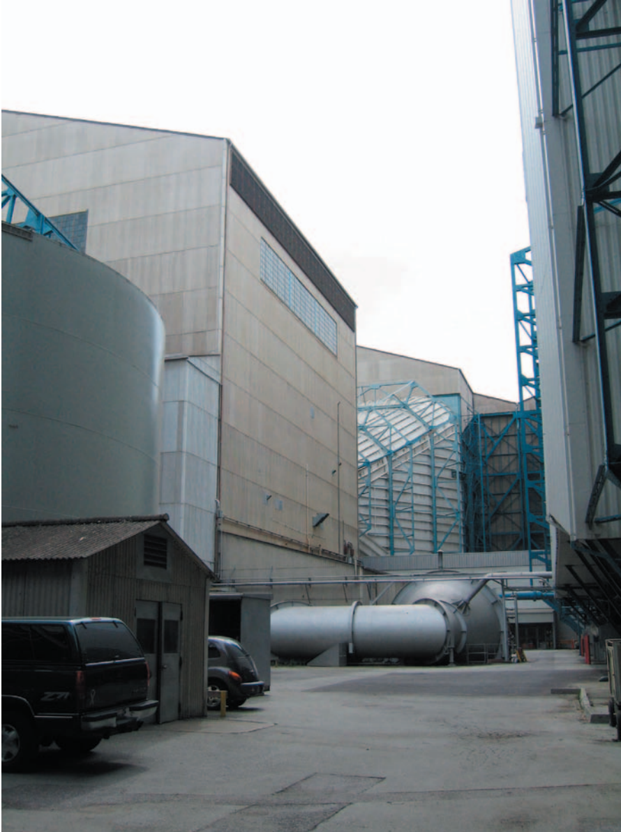
Figure 24. Courtyard looking south
