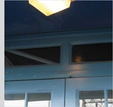
Illustration 4. 2-lite transom at north elevation of Wind Tunnel is a significant feature. (Source: ARG, October 2006)
