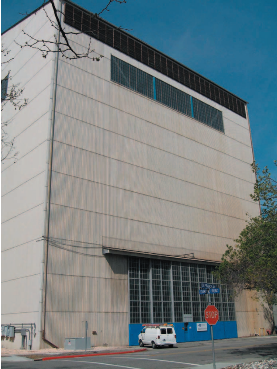
Figure 18. East facade Tunnel entry
