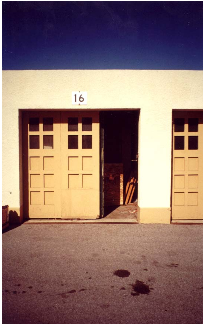
Man Door within Sliding Garage Door Building 21 & 22 Moffett Field
