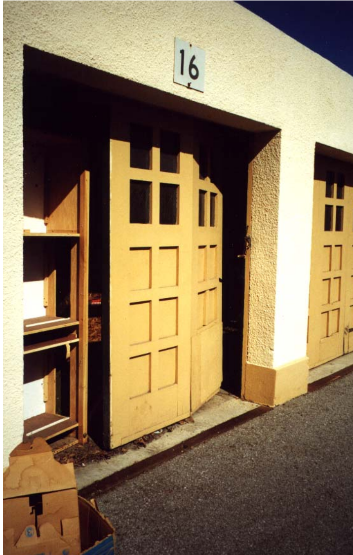
Sliding Garage Door Building 21 & 22 Moffett Field
