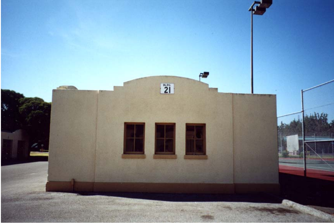
North Facade Building 21 Moffett Field
