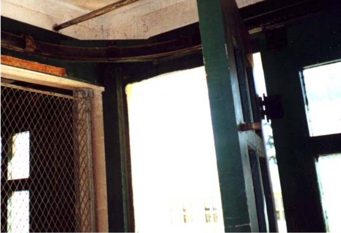
Detail of Door Track Building 21 & 22 Moffett Field
