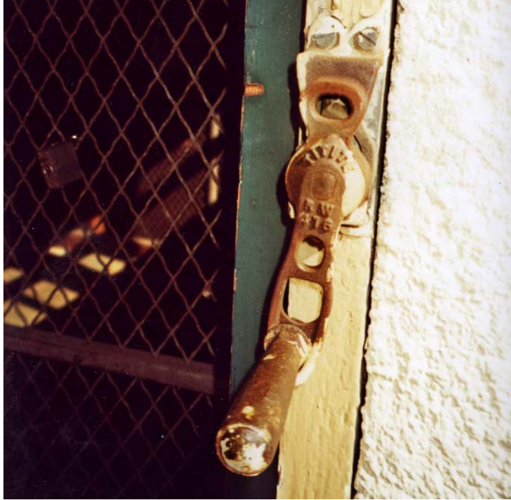
Detail of Door Hardware Building 21 & 22 Moffett Field
