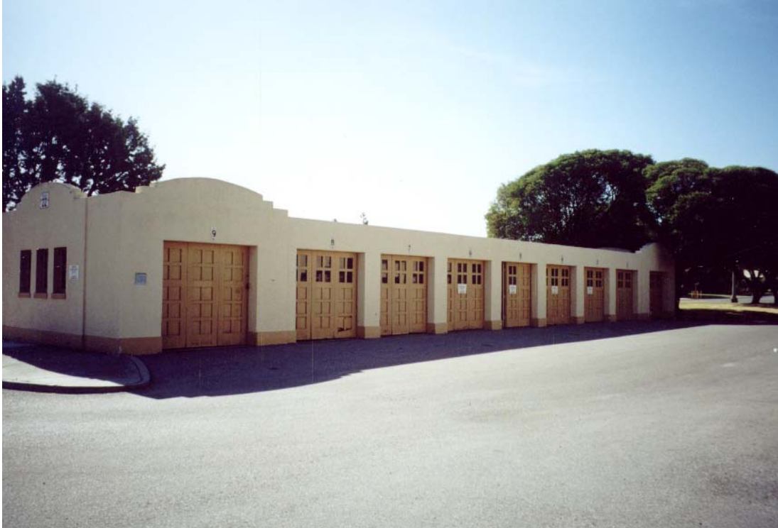
West Facade Building 22 Moffett Field
