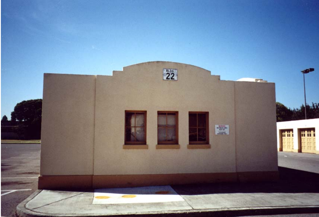
North Facade Building 22 Moffett Field
