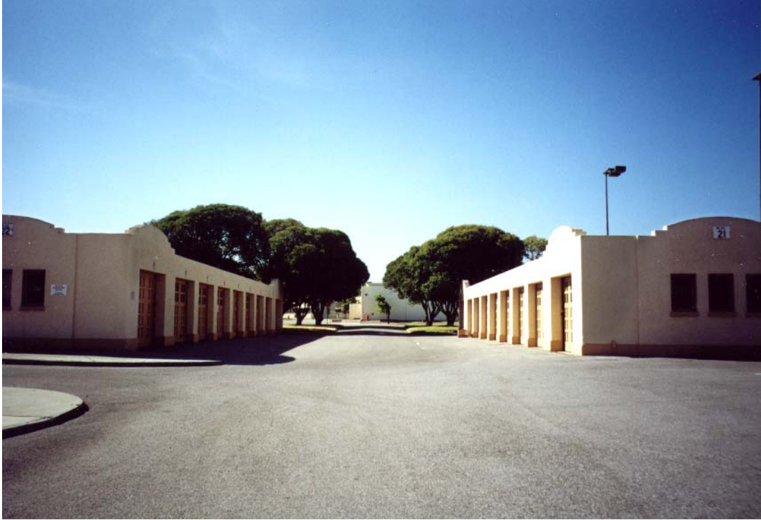
Buildings Viewed from the North Building 21 & 22 Moffett Field
