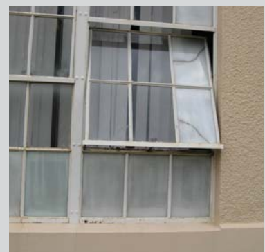
Illustration 3: Multi-lite metal sash windows with operable awning segments are a significant feature. (Source: ARG, October 2006)
