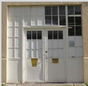
Illustration 5: Multi-lite metal doors are a significant feature. (Source: ARG, October 2006)
