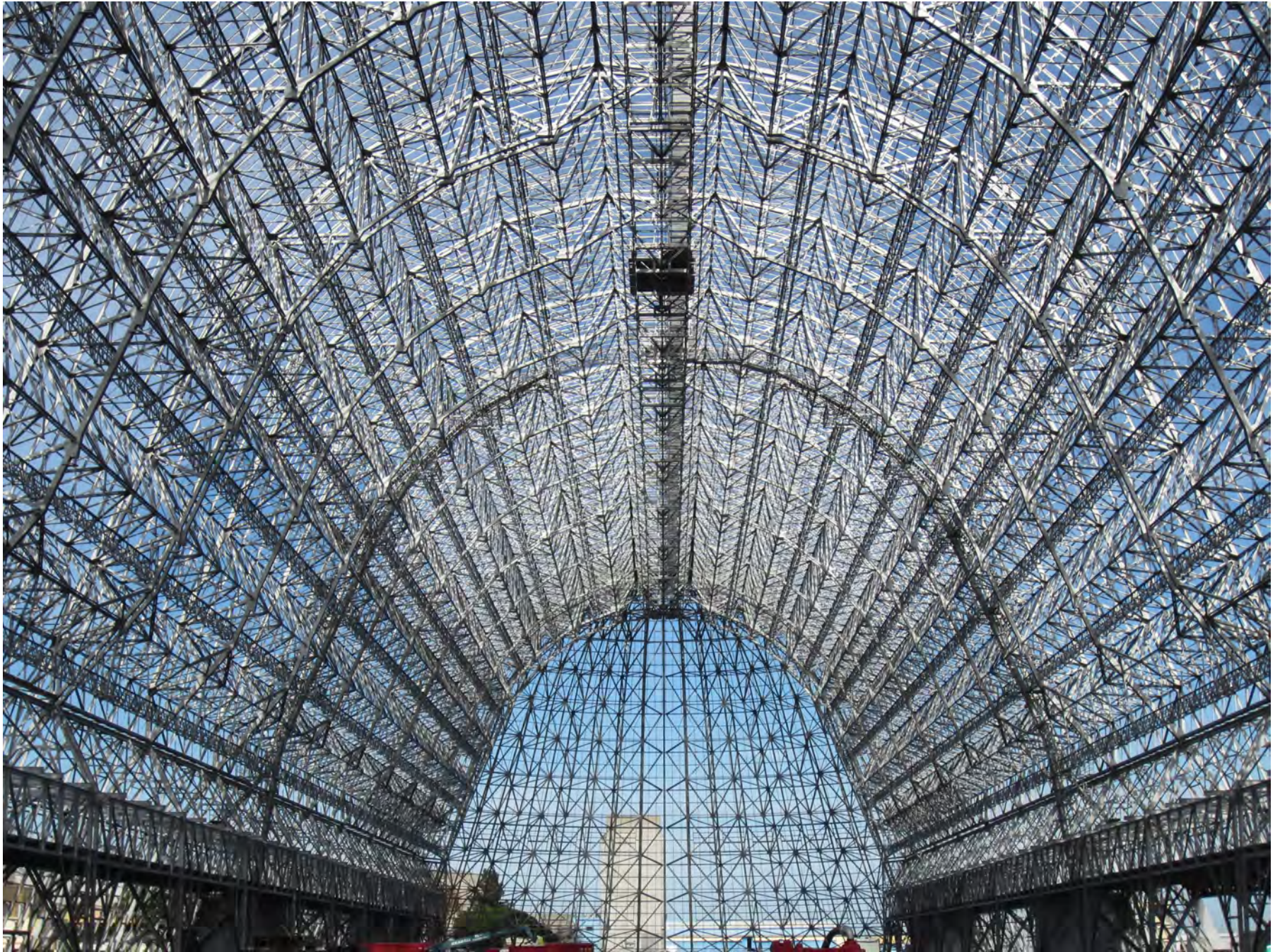
HANGAR 1 INTERIOR, BUILDING SKIN REMOVED
