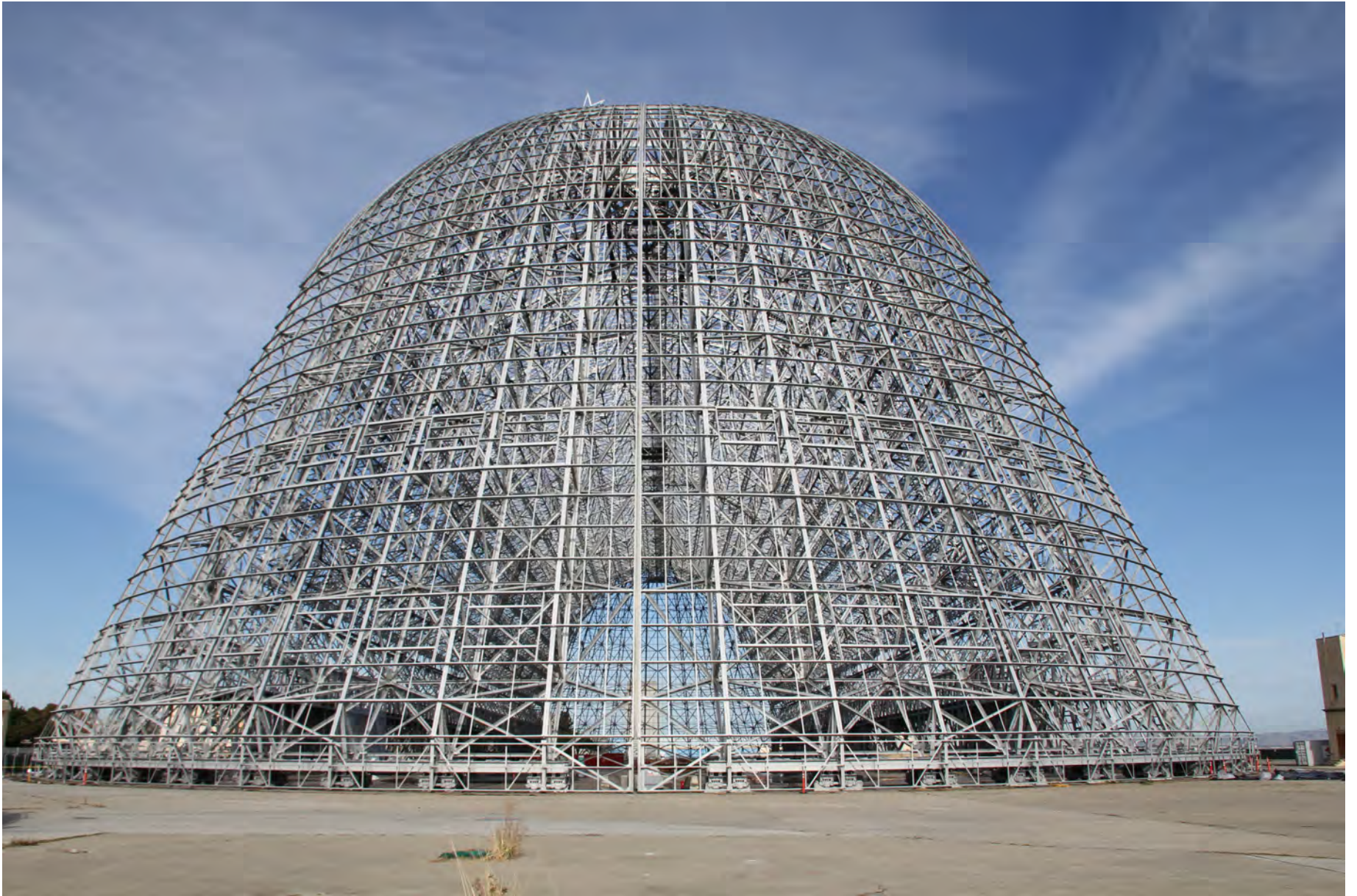
HANGAR 1 END VIEW, BUILDING SKIN REMOVED
