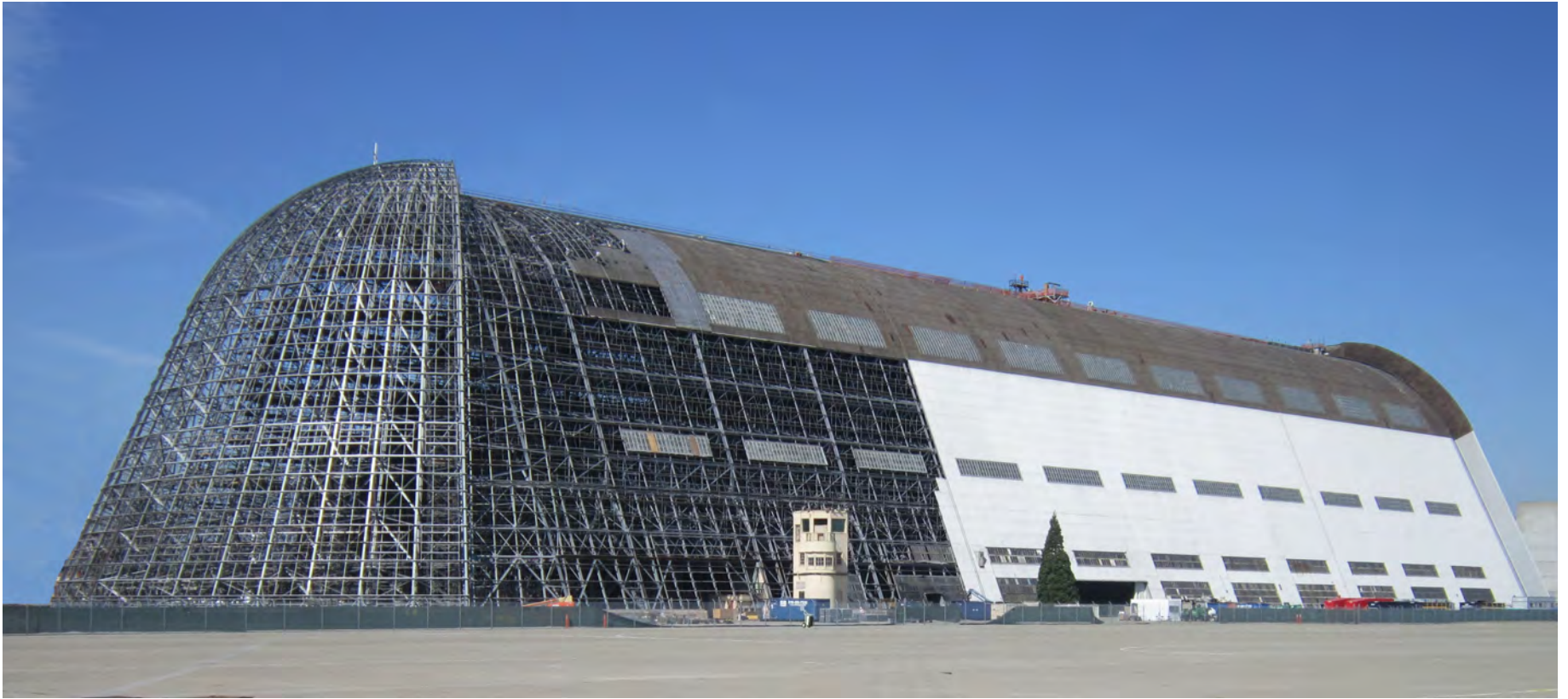
HANGAR 1 SIDE VIEW, BUILDING SKIN PARTIALLY REMOVED
