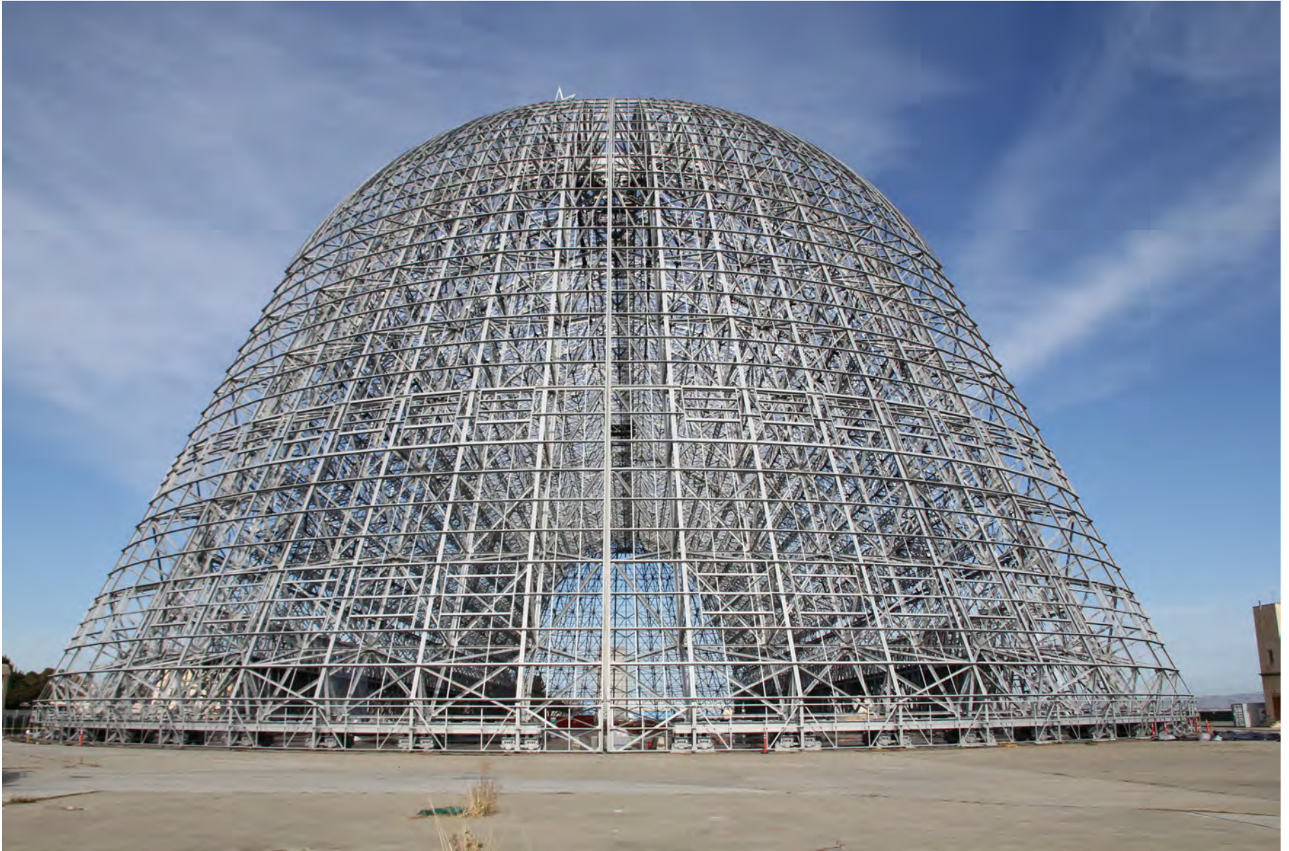
HANGAR 1 END VIEW, BUILDING SKIN REMOVED
