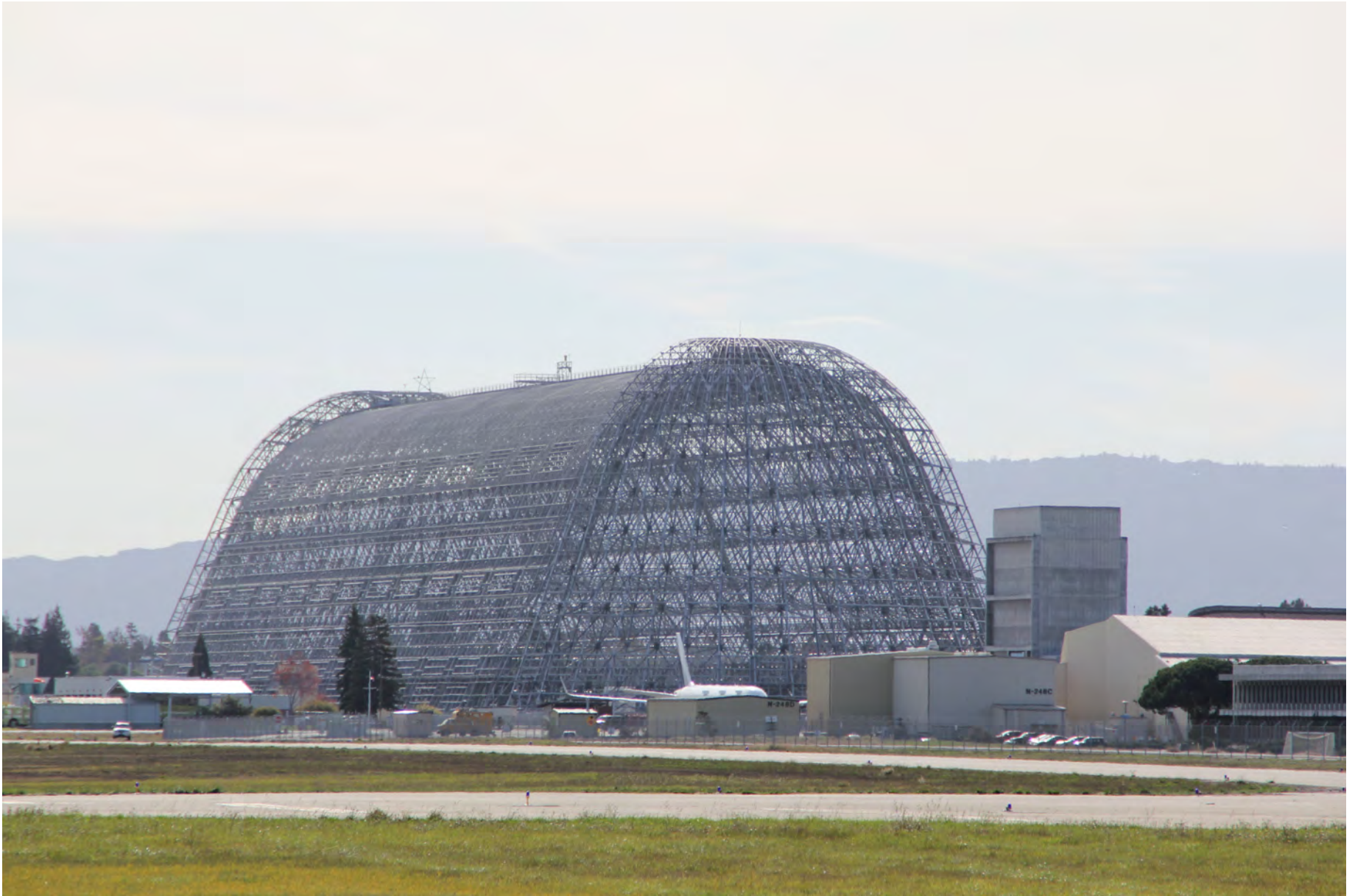
HANGAR 1 SIDE AND END VIEW, BUILDING SKIN REMOVED
