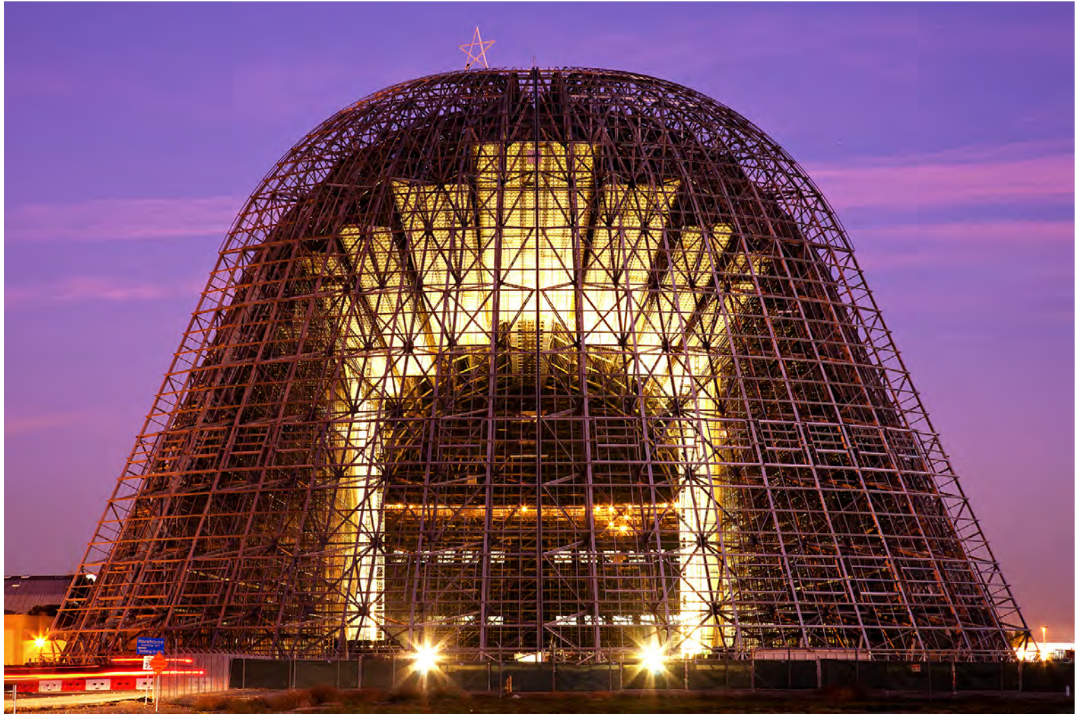
HANGAR 1 END VIEW, ILLUMINATED, BUILDING SKIN REMOVED
