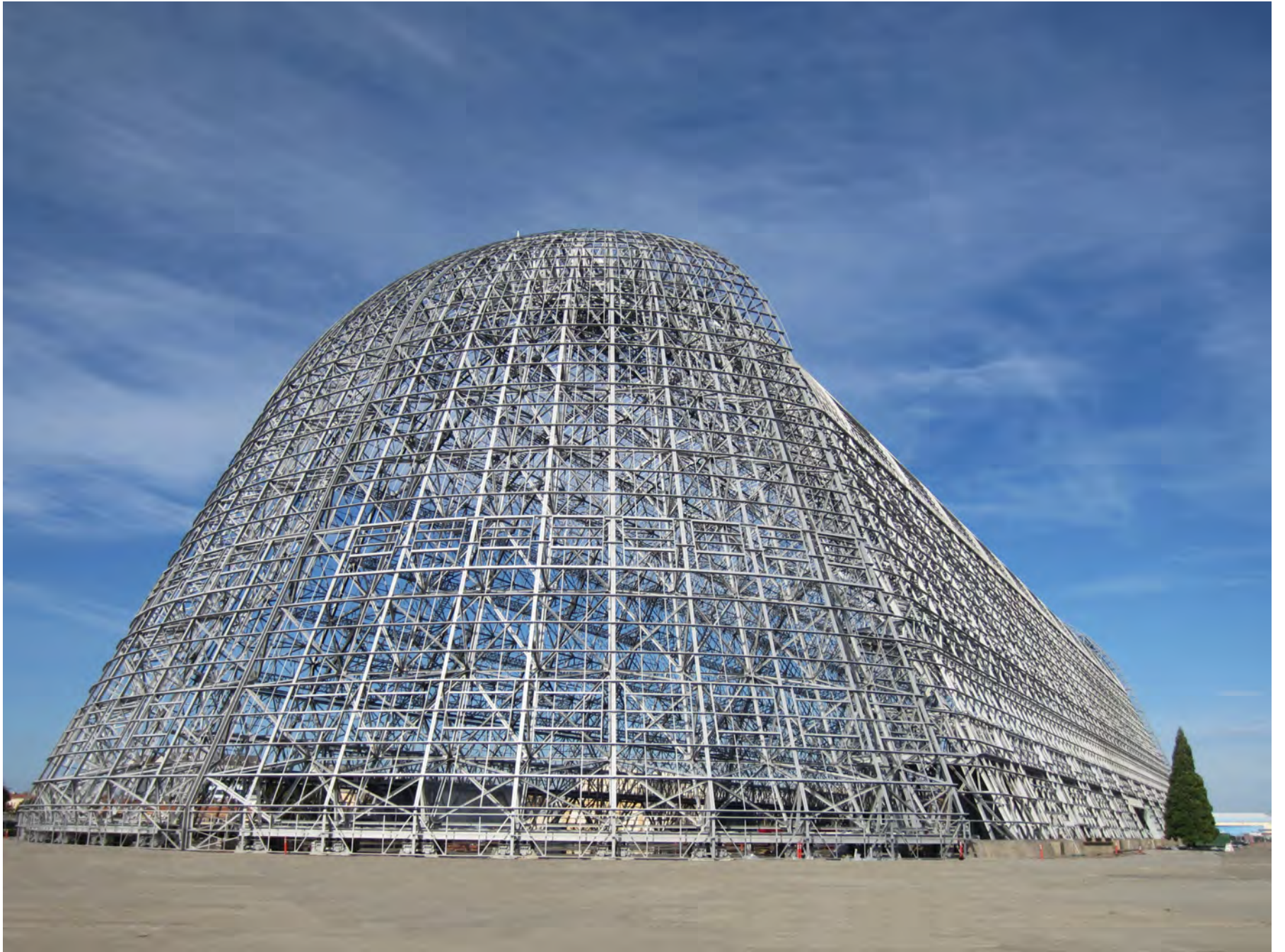
HANGAR 1 END VIEW, BUILDING SKIN REMOVED
