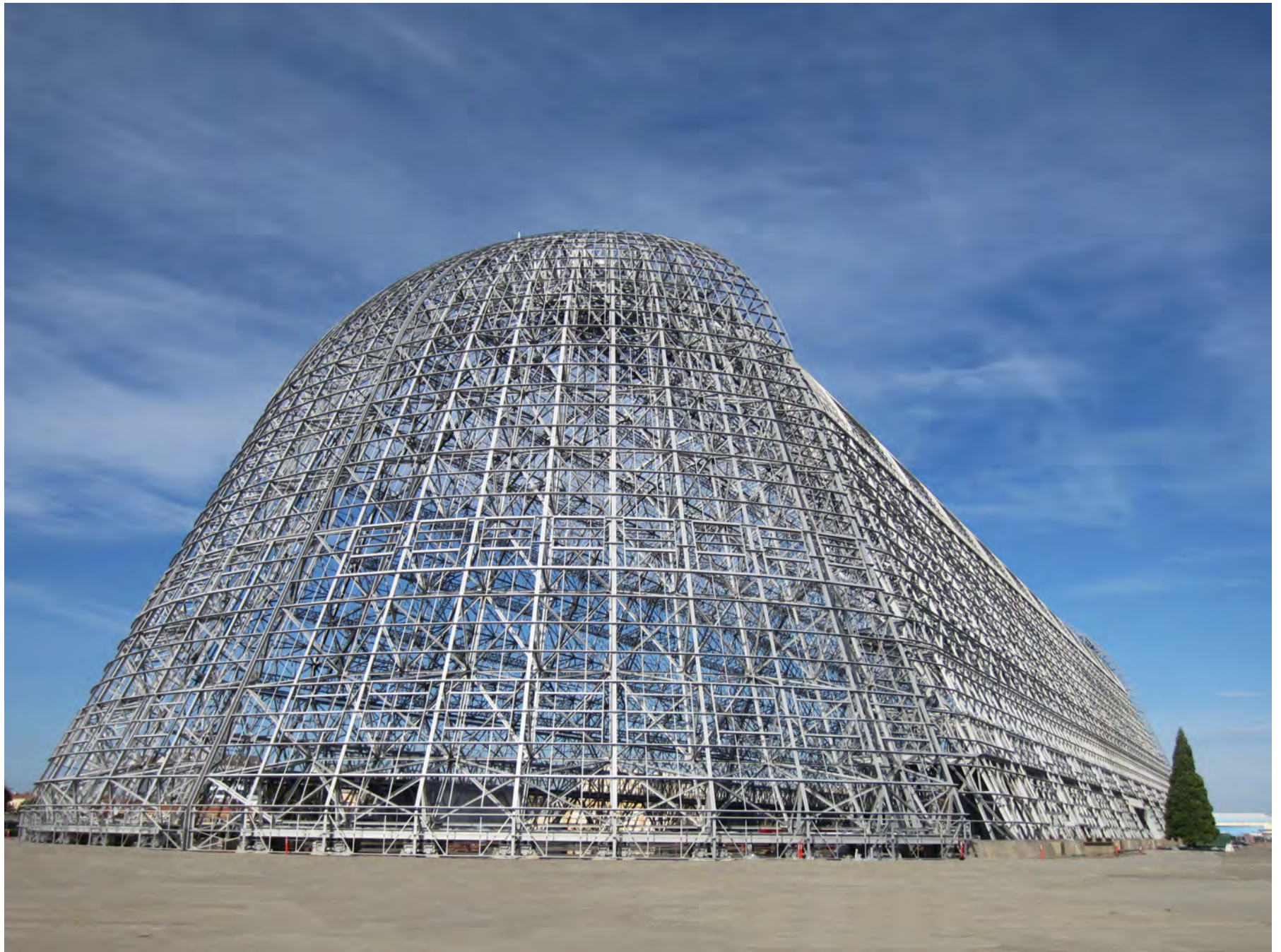
HANGAR 1 END VIEW, BUILDING SKIN REMOVED
