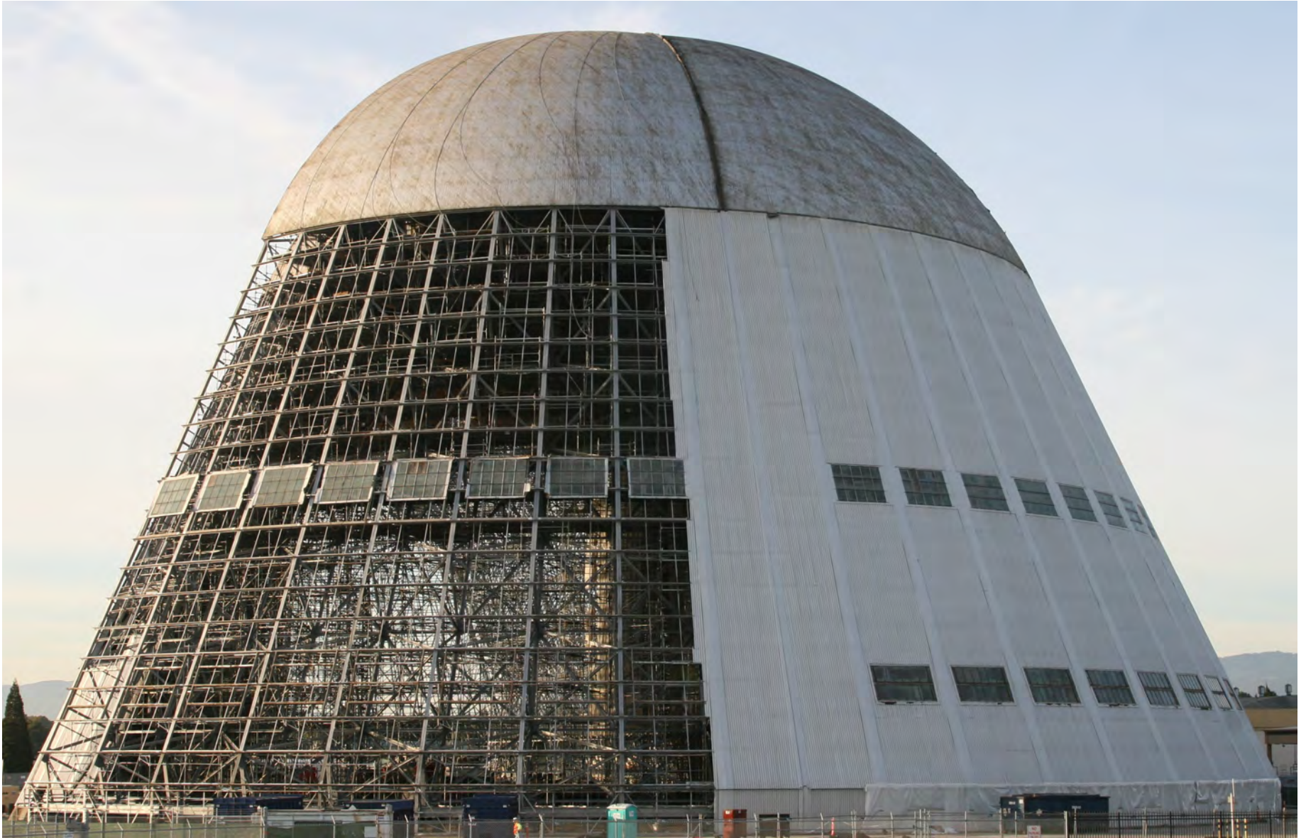
HANGAR 1 END VIEW, BUILDING SKIN PARTIALLY REMOVED
