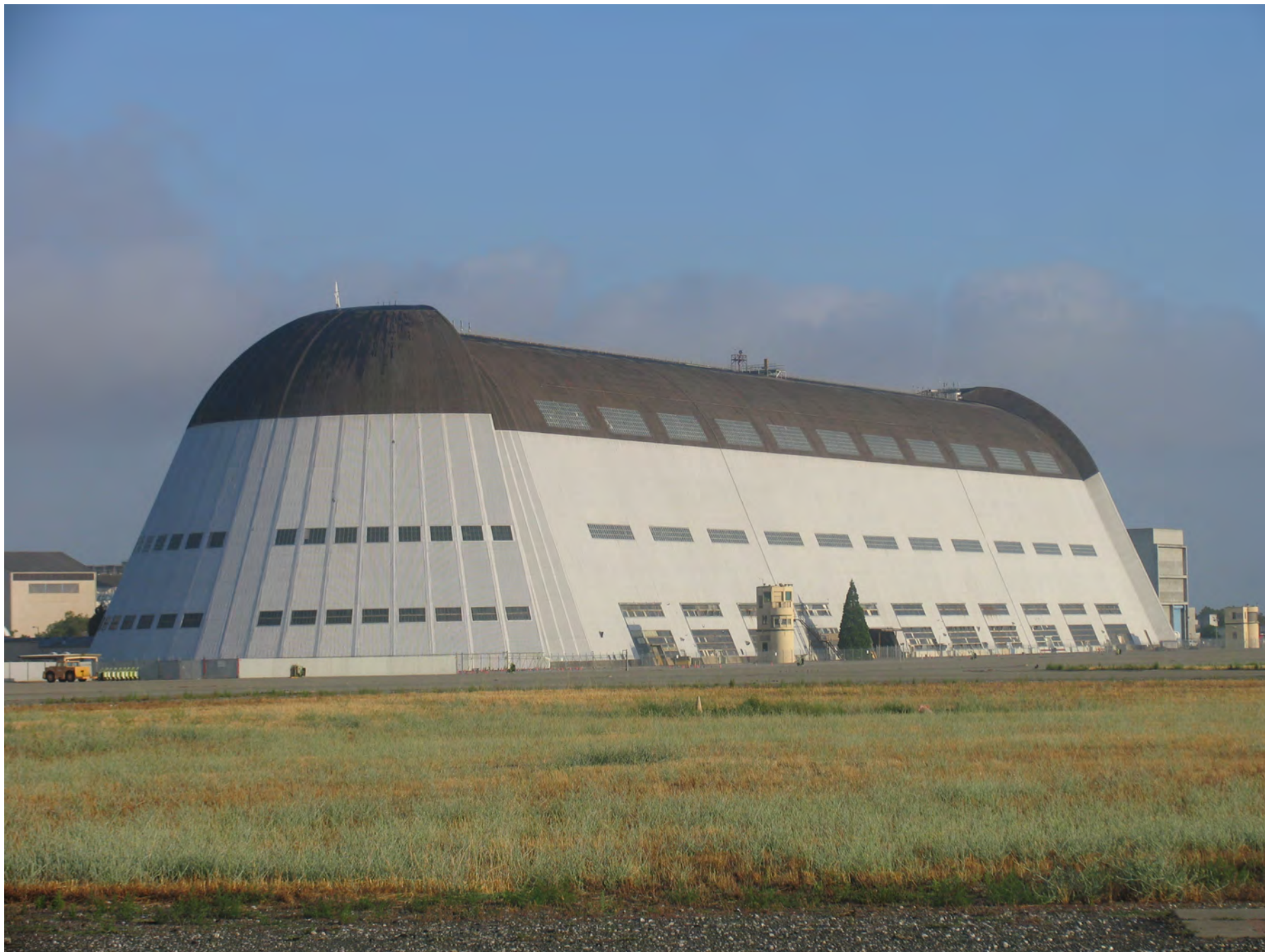
HANGAR 1 SIDE AND END VIEW, BUILDING SKIN INTACT
