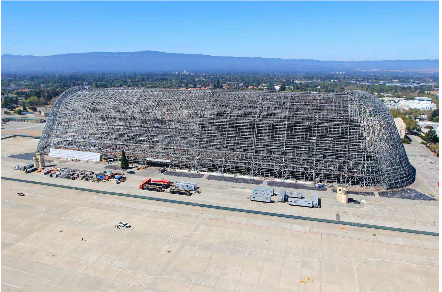
HANGAR 1 SIDE VIEW, BUILDING SKIN REMOVED
