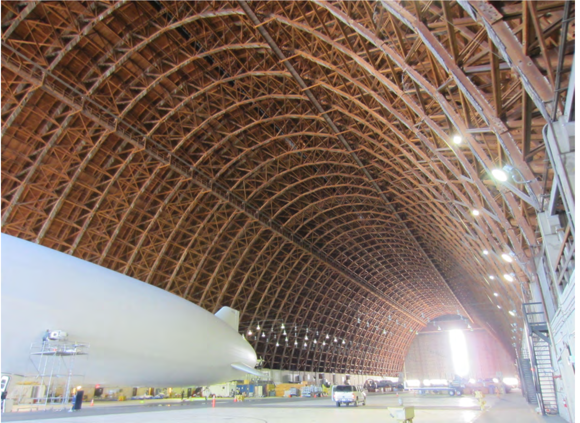
HANGAR 2 INTERIOR VIEW
