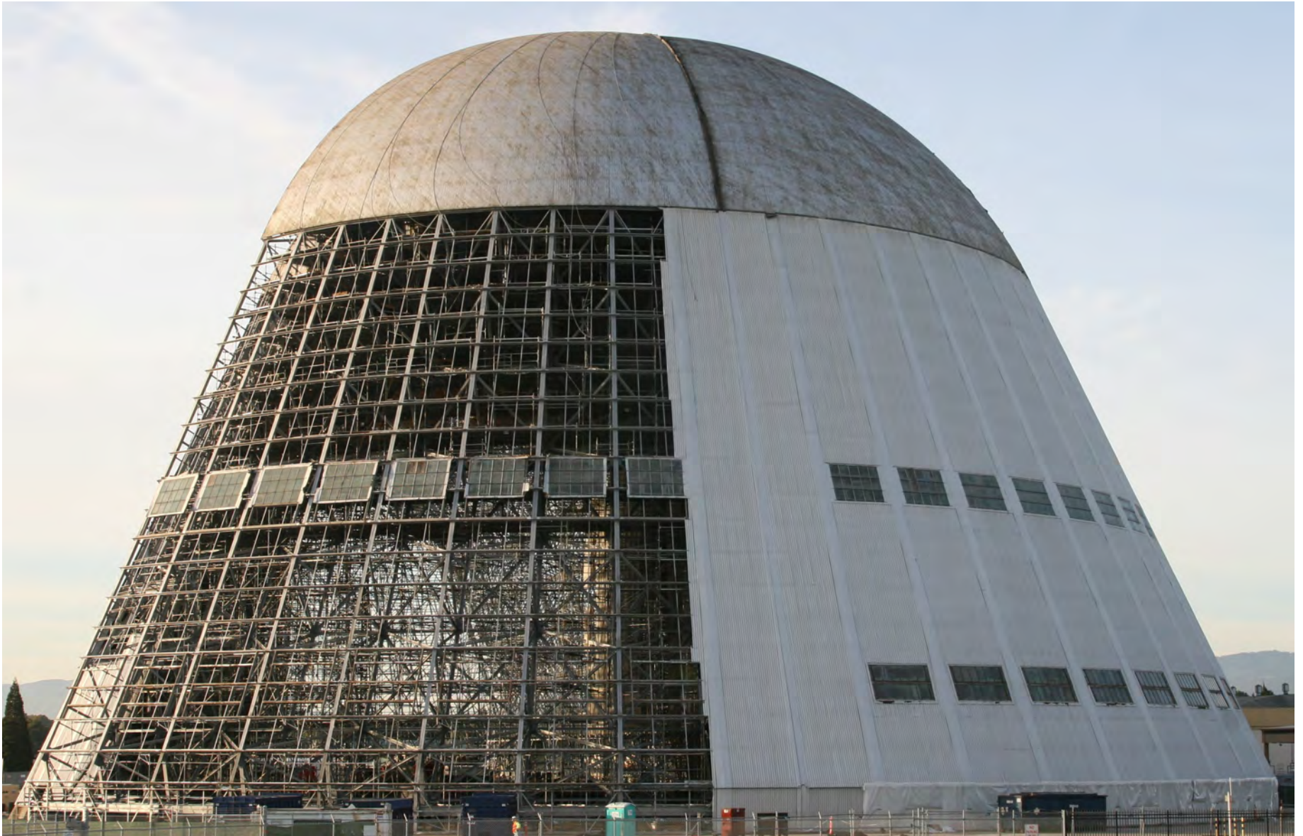
HANGAR 1 END VIEW, BUILDING SKIN PARTIALLY REMOVED
