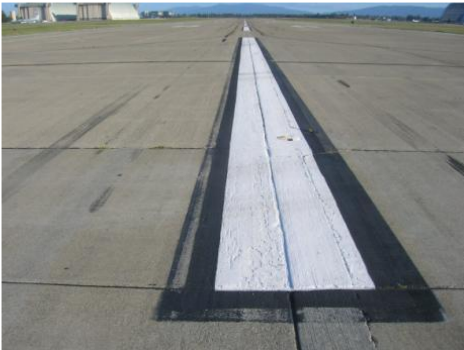
Photo 6. Runway 14L, Section R02CA, Overview
