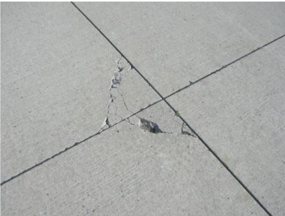
Photo 18. East Taxiway, Section T04A, High Severity Corner Spall.
