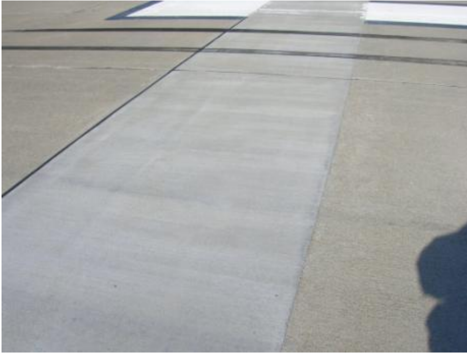
Photo 7. Runway 14L, Section R03C, Low Severity Large Patch.
