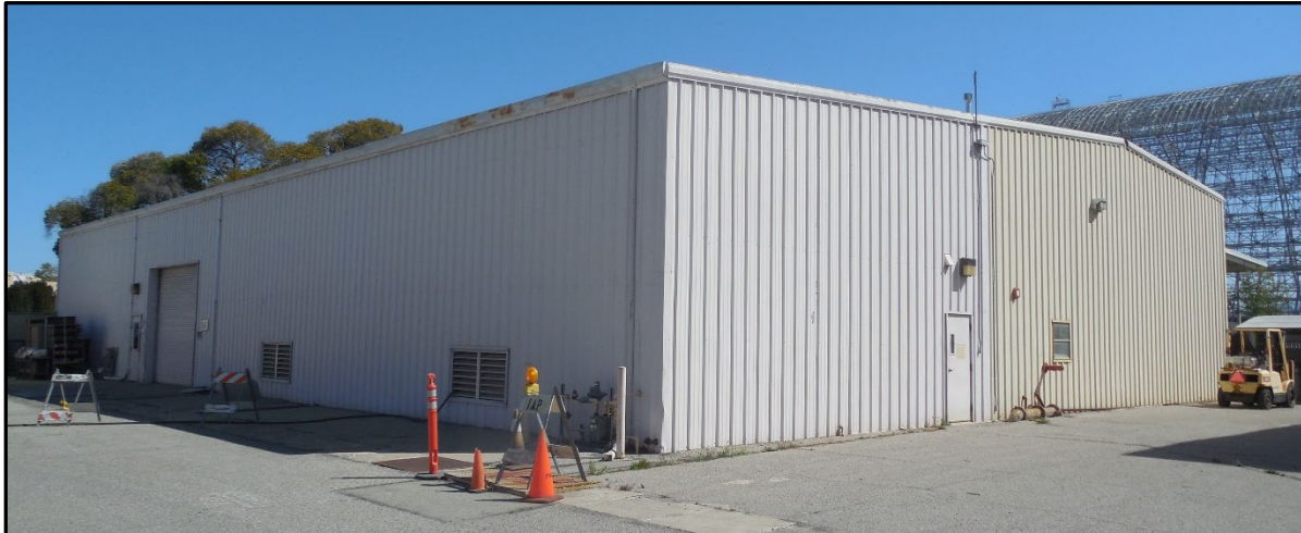
Figure 9. Building 567 west and south elevations.
