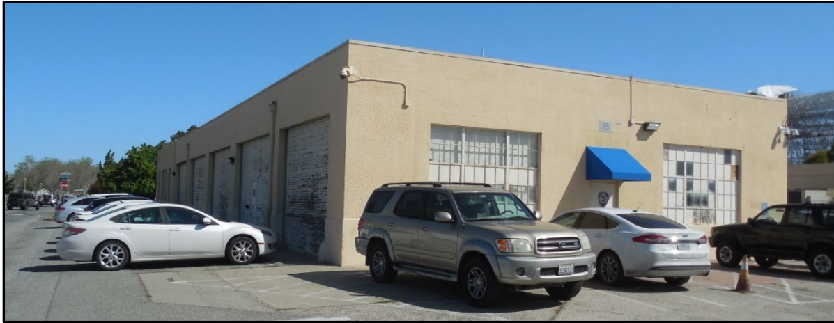
Figure 5. Building 15 west and south elevations.
