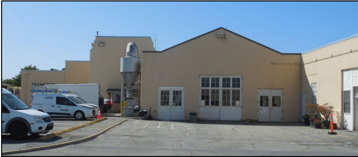
Figure 7. Building 16 north elevation.
