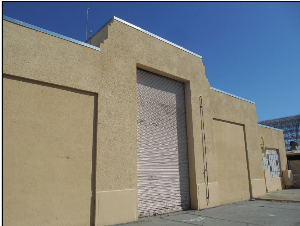
Figure 8. Building 16 south elevation.
