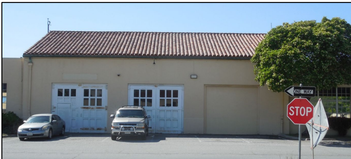
Figure 4. Building 15 north elevation center.
