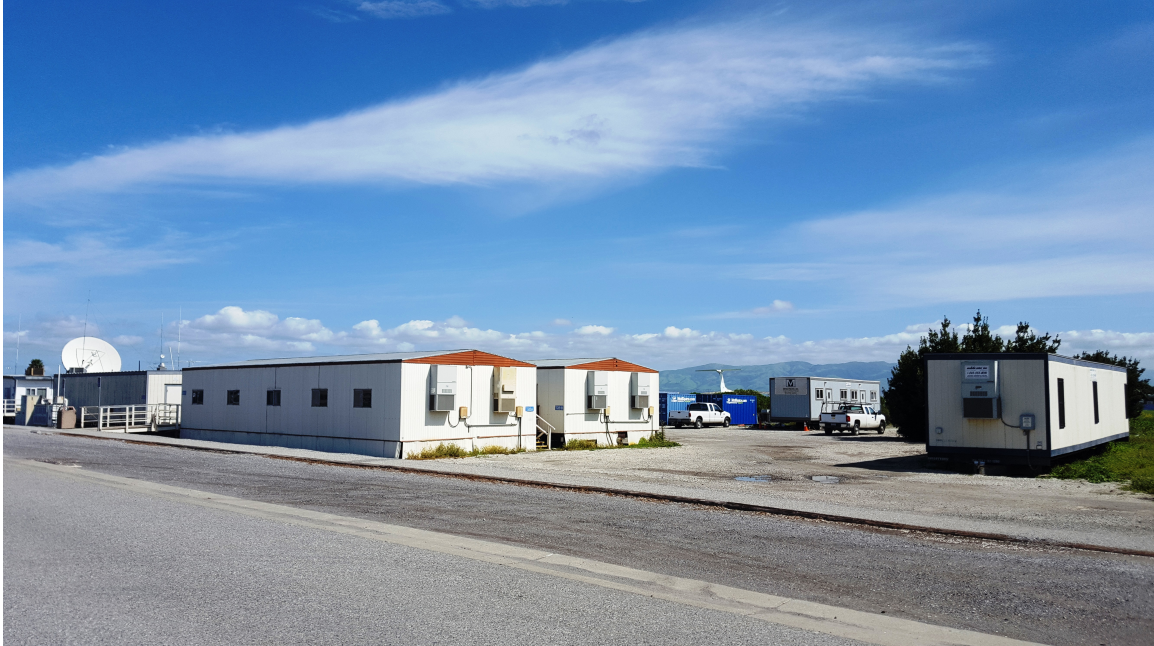
Plate 3. MSF site, view facing northeast from DeFrance Avenue (TA28A and TA28B at left).
