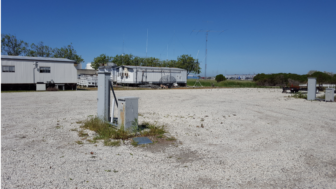
Plate 5. MSF site, view facing northwest.
