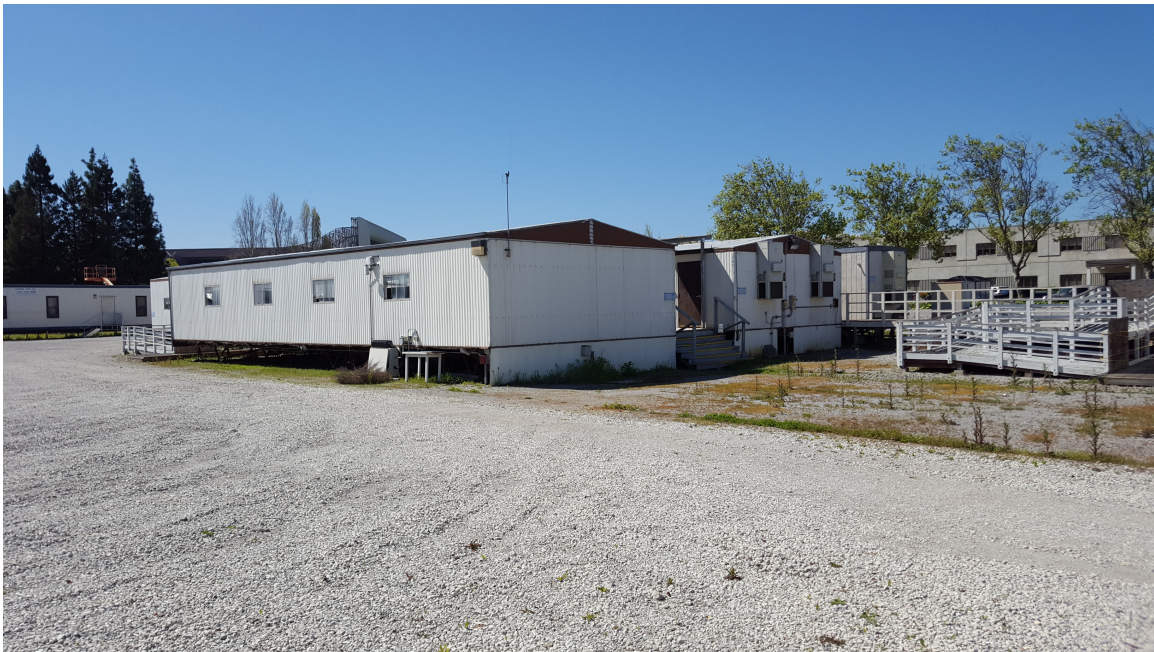
Plate 4. MSF site, view facing southwest (opposite view of TA28A and TA28B in foreground at center, Building N-255 in background at right).
