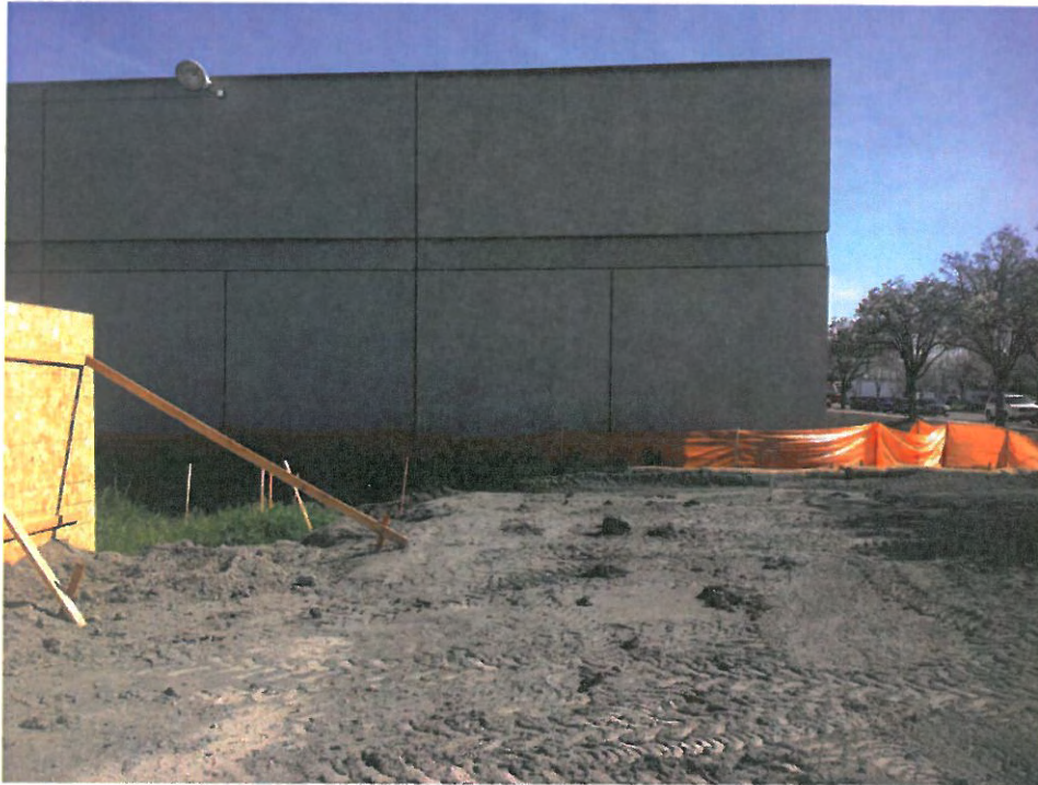
Plate 1. Project site, view facing east (Building N255 in background).
