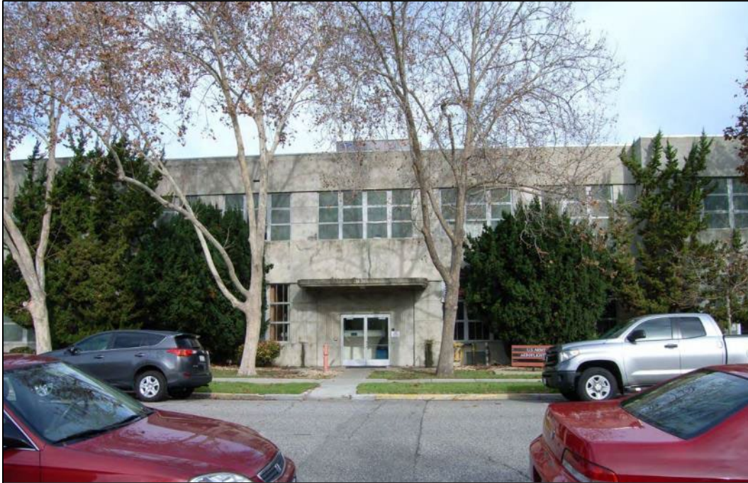
Photograph 2. Primary entry in Building N215 on southern-facing façade, view to north.
