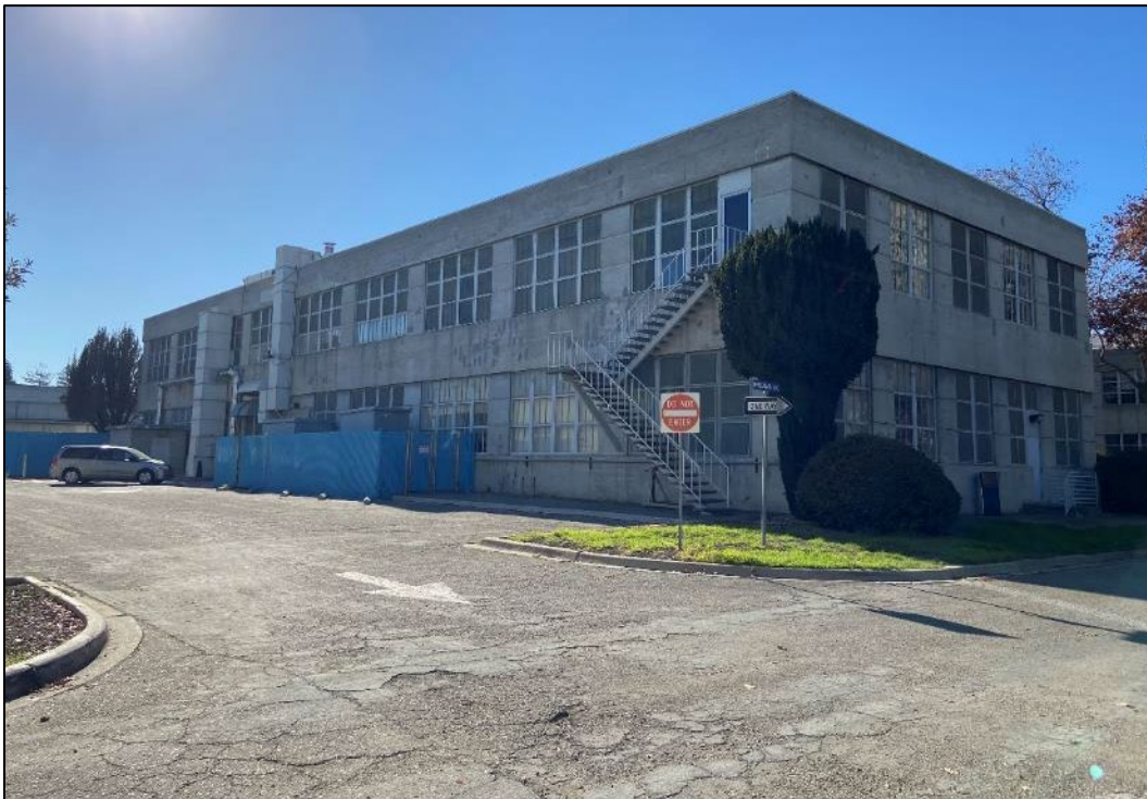
Photograph 7. North and east sides of Building N203, view facing southwest.
