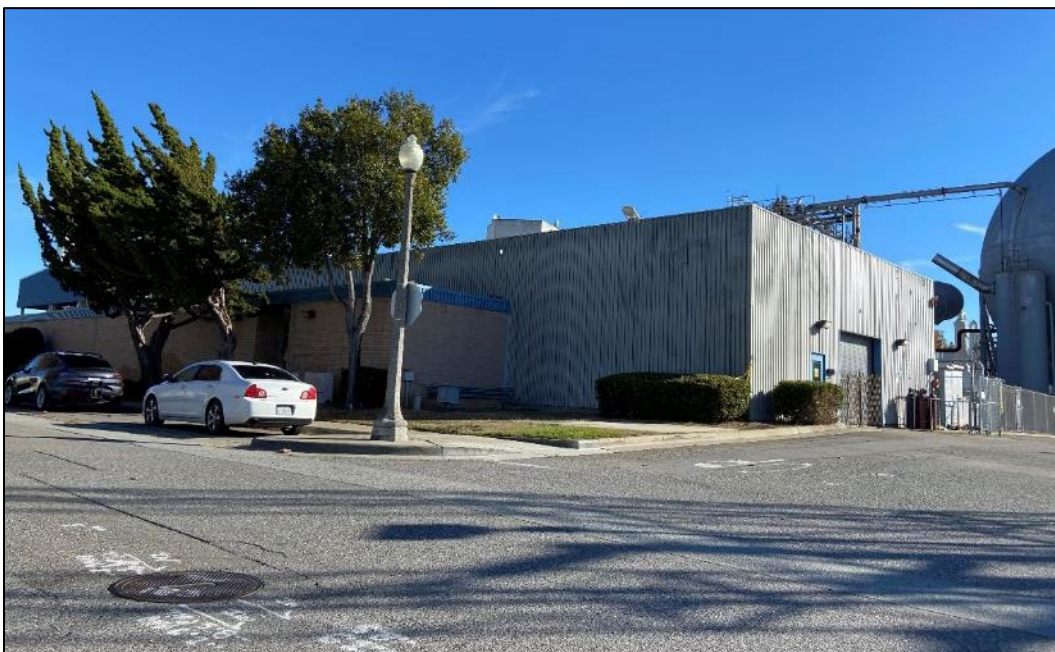
Photograph 16. North and west sides of Building N238, view to southeast.
