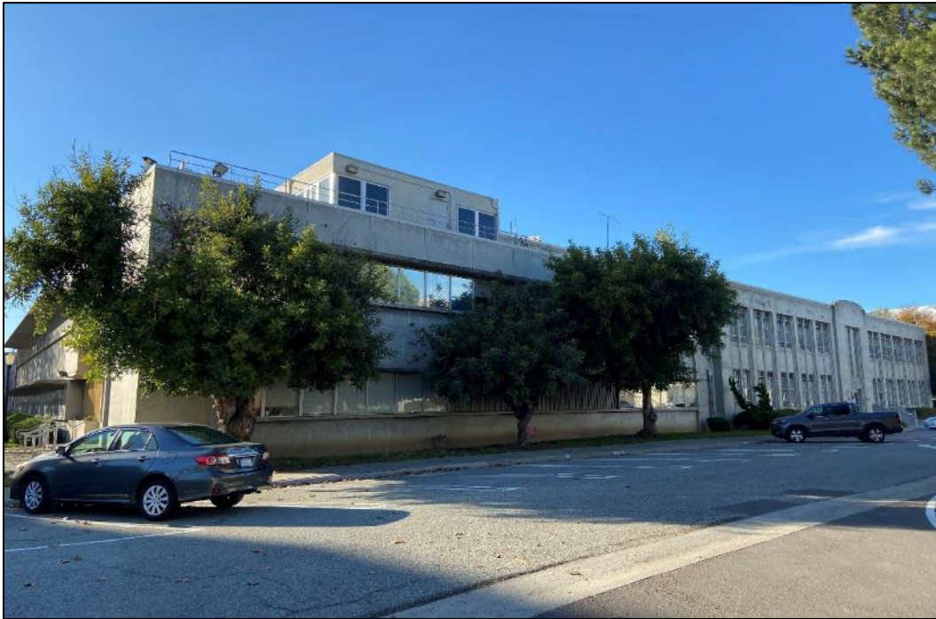
Photograph 8. South side and eastern-facing façade of Building N210. The 1960-constructed addition is on the left, view to northwest.
