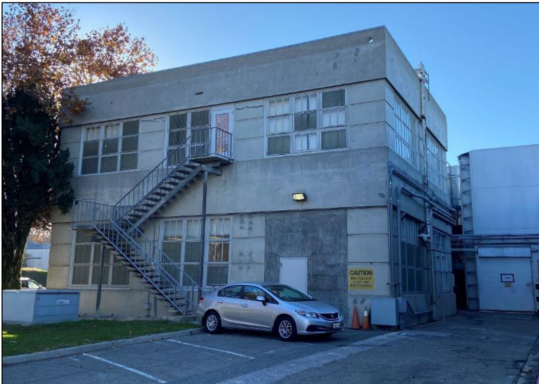
Photograph 3. East side of Building N215, view to west.
