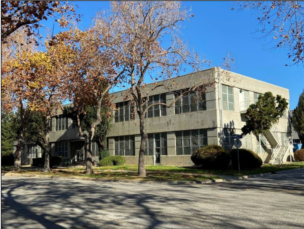
Photograph 6. Western-facing façade of Building N203, view facing northeast.
