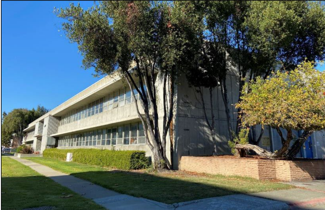
Photograph 10. East and south sides of Building N230, view to northwest.
