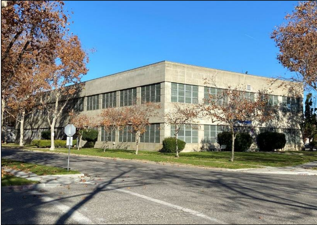
Photograph 4. West and south sides of Building N220, view to northeast.
