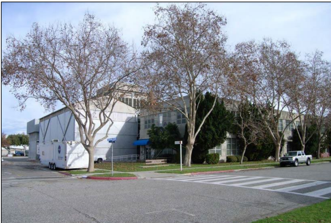
Photograph 1. West and south sides of Building N215, view to northeast.
