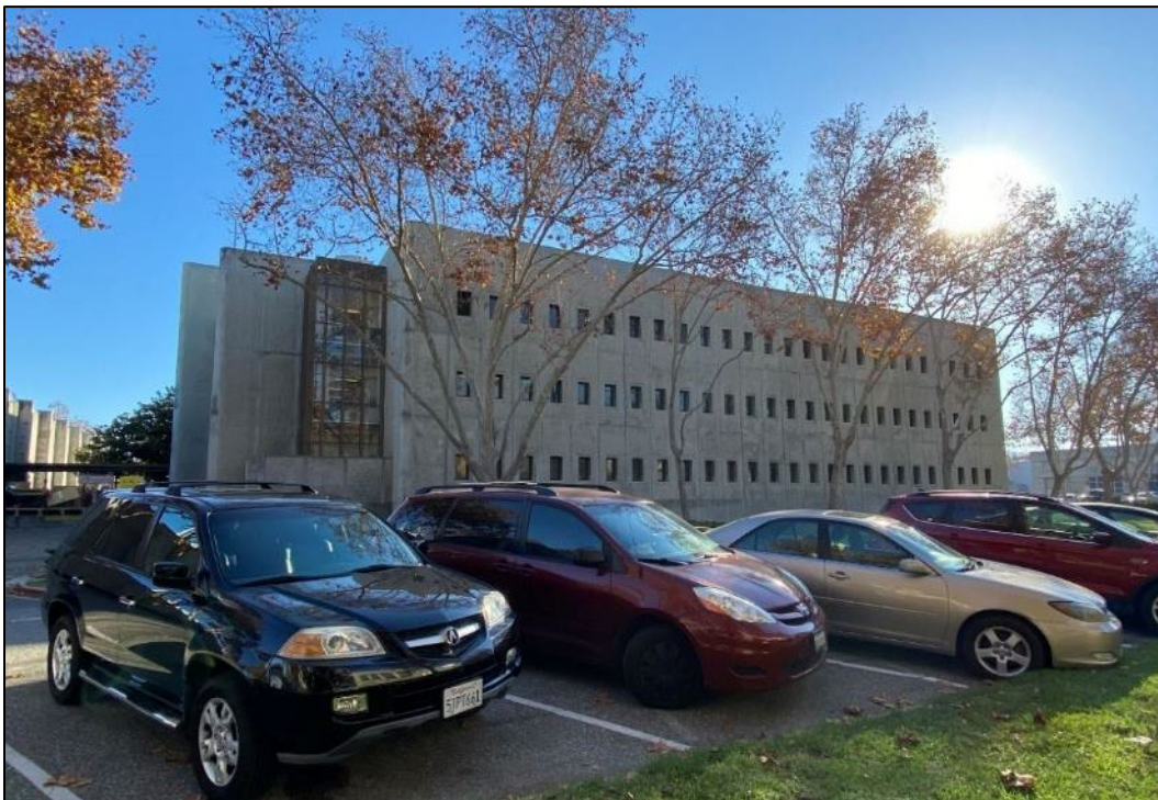
Photograph 18. South side of Building N239, view facing north.
