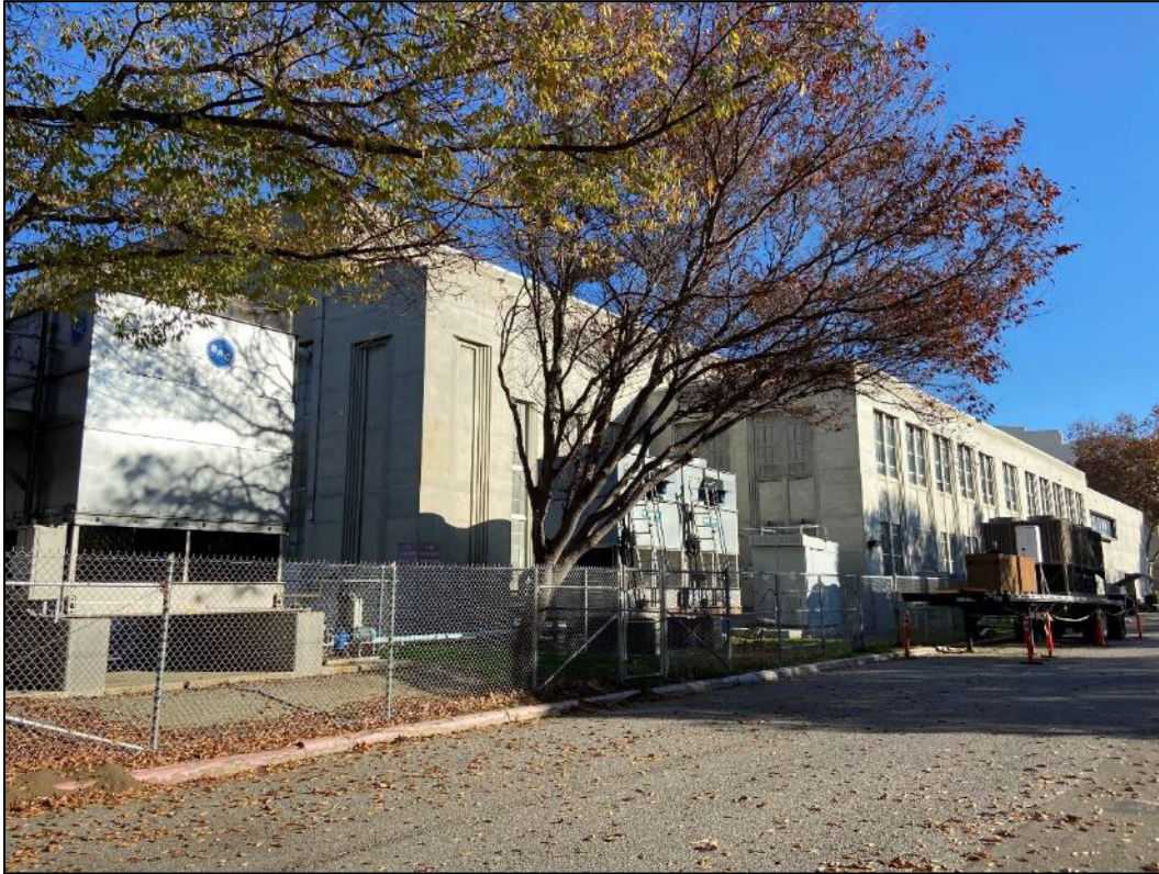
Photograph 9. North and west sides of Building N210, view to southeast.
