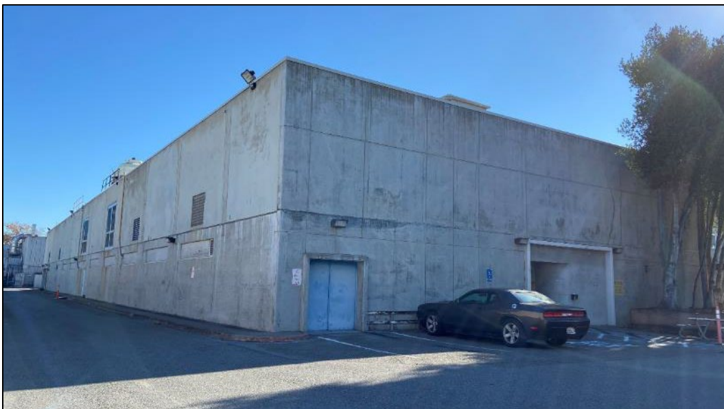
Photograph 11. West and south sides of Building N230, view to southeast.
