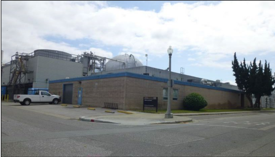
Photograph 15. North and east sides of Building N238, view to southwest.
