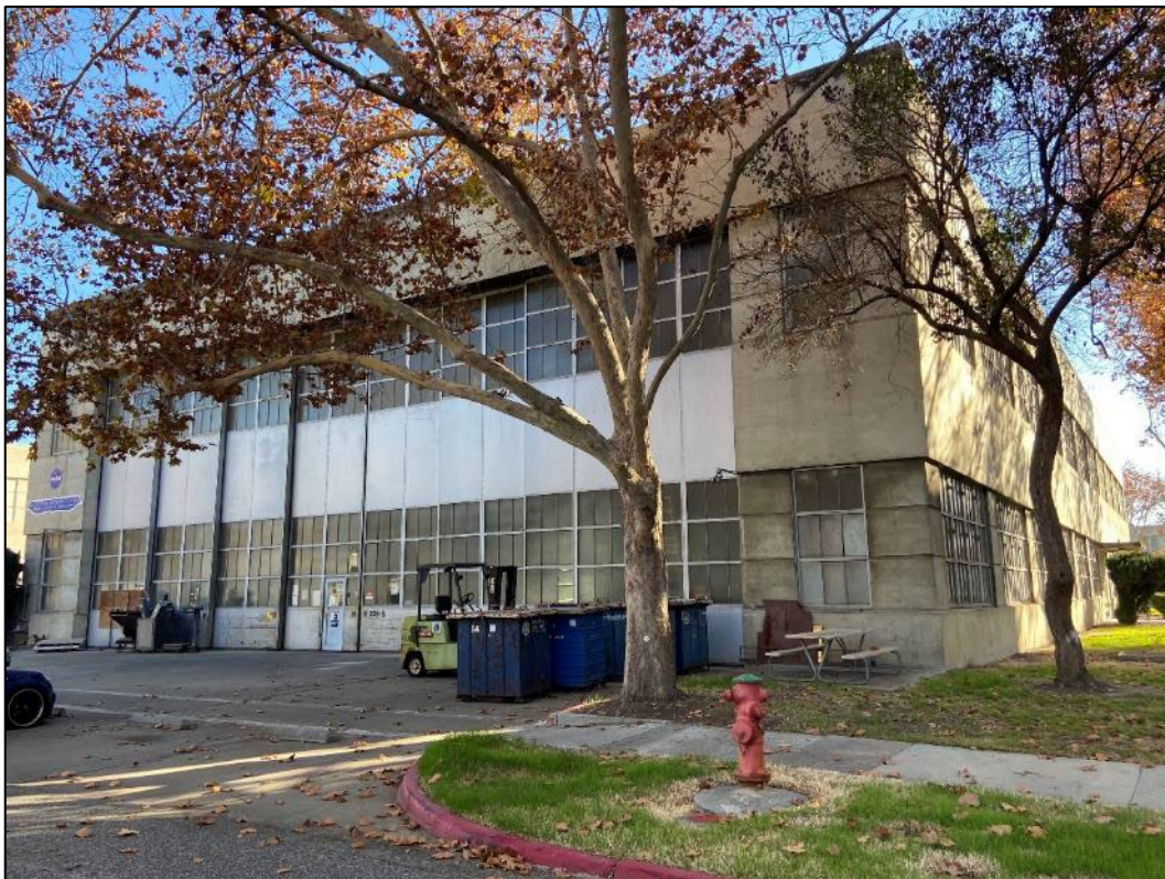
Photograph 5. North and west sides of Building N220, showing hangar door, view to southeast.
