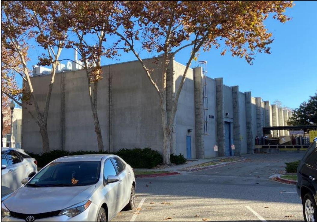
Photograph 22. North and west sides of Building N239A, view facing southeast.
