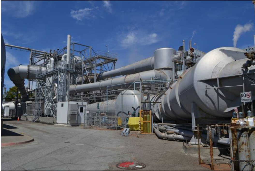
Photograph 13. SWS, southwest side of the Arc Jet Complex, view to northeast.
