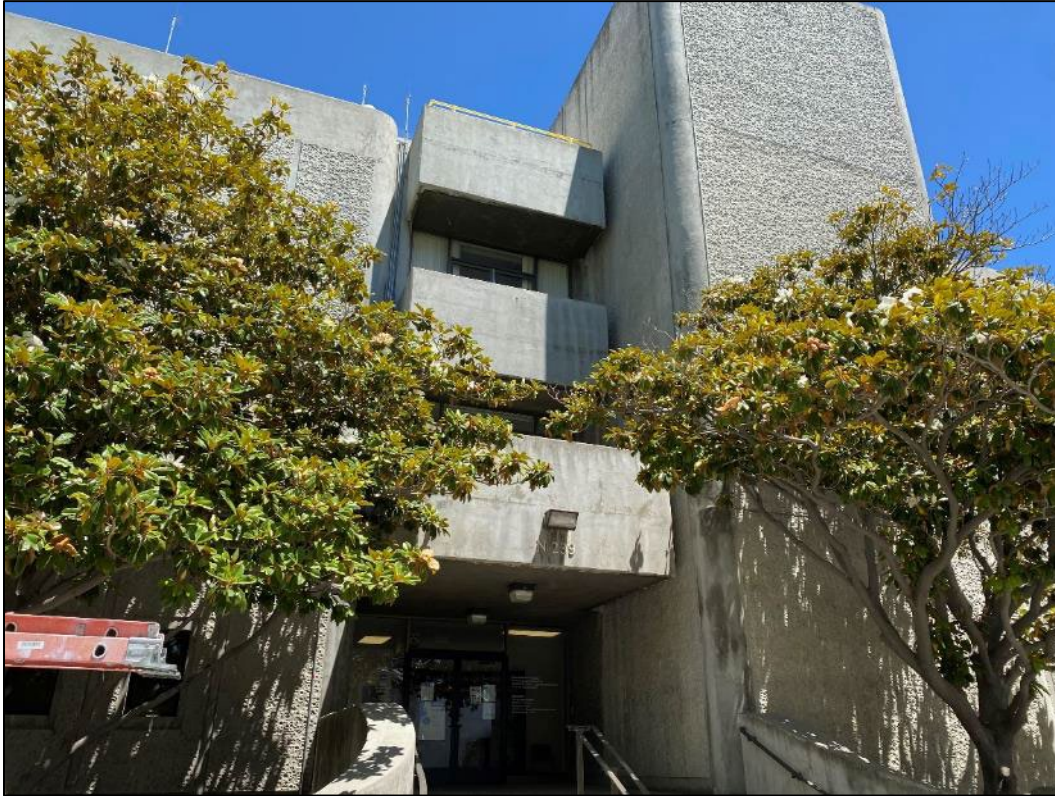
Photograph 19. Primary entry on west side of Building N239, view facing east.
