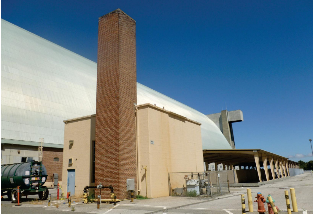
Plate 3. Building 55, view facing northwest
