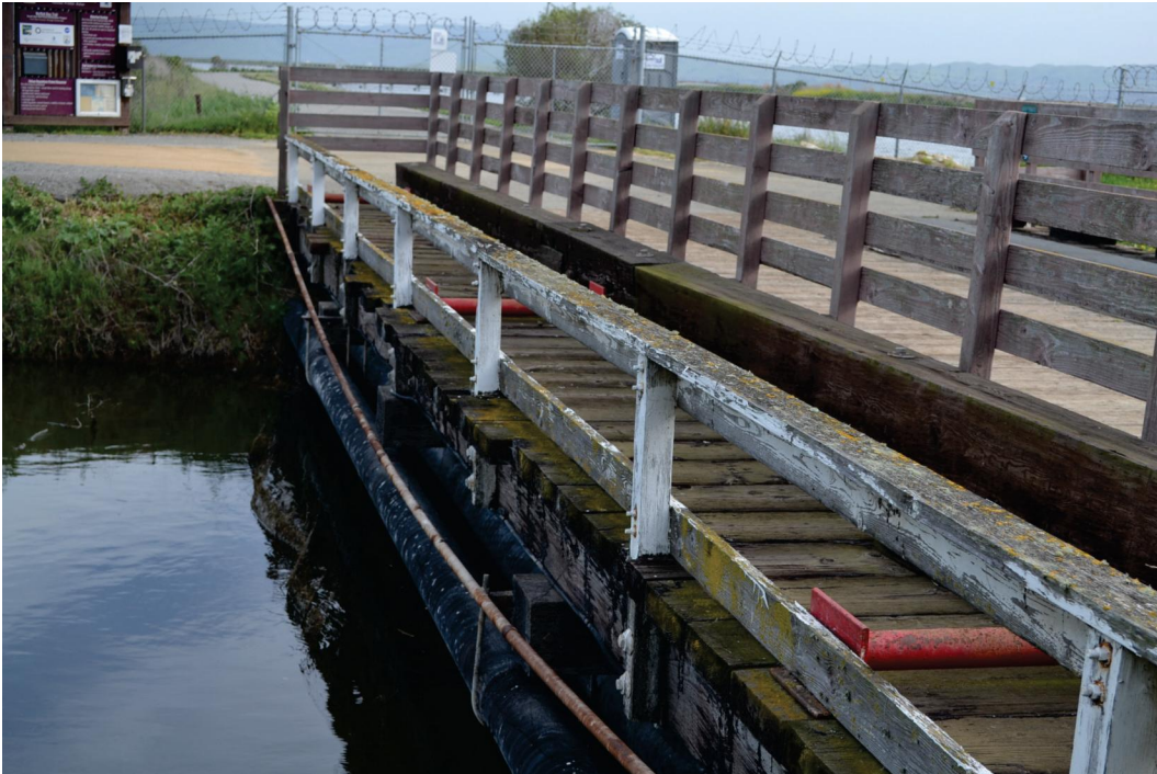
Plate 10. Building 169 (Bridge), view facing northeast
