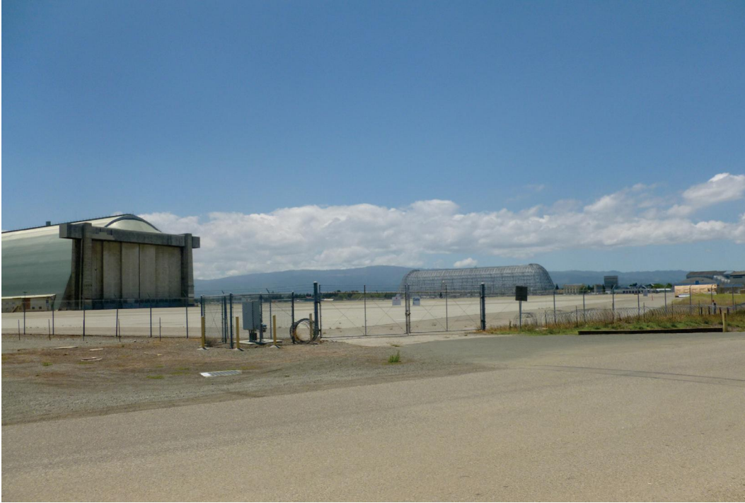
Plate 6. MF1002, apron adjacent to Hangars 2 and 3, view facing southwest
