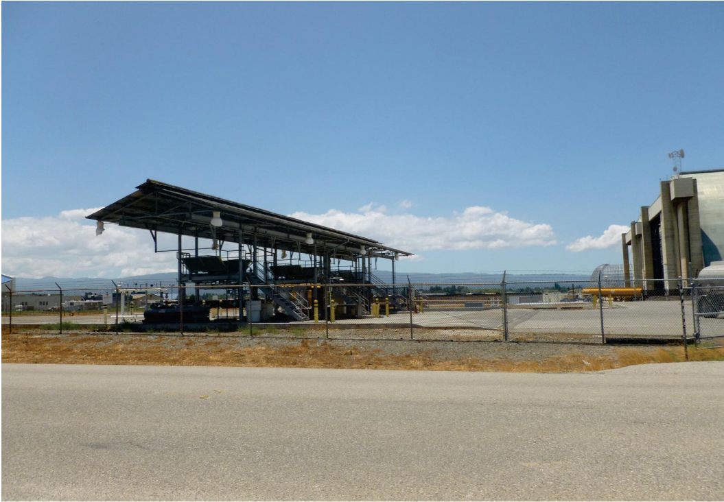
Plate 9. Building 141, view facing west
