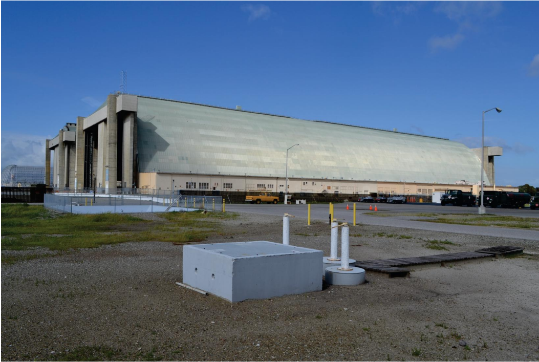
Plate 2. Hangar 3 (Hangar 2 behind), view facing northwest from Building 141
