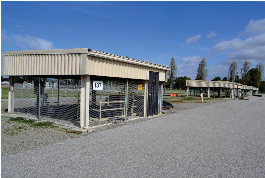
Plate 8. Sheds housing UST controls (Buildings 137–140), view facing north
