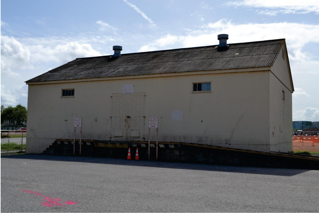
Plate 4. Building 69, view facing southeast
