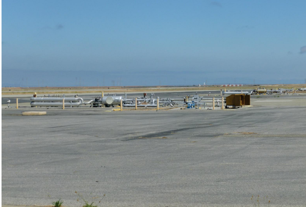
Plate 13. Aboveground fueling pits infrastructure (hydrants removed), view facing north
