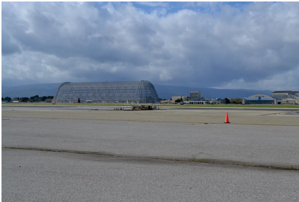
Plate 7. MF1016, taxiway pavement, view facing southwest
