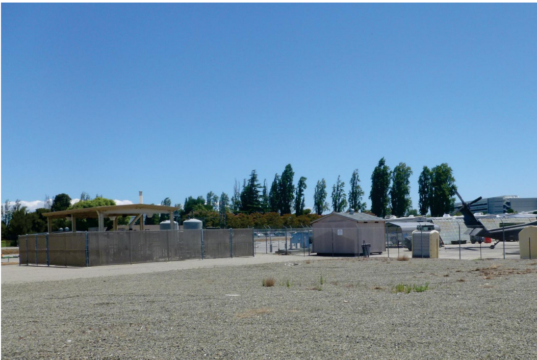
Plate 5. Building 439, at left, view facing southeast
