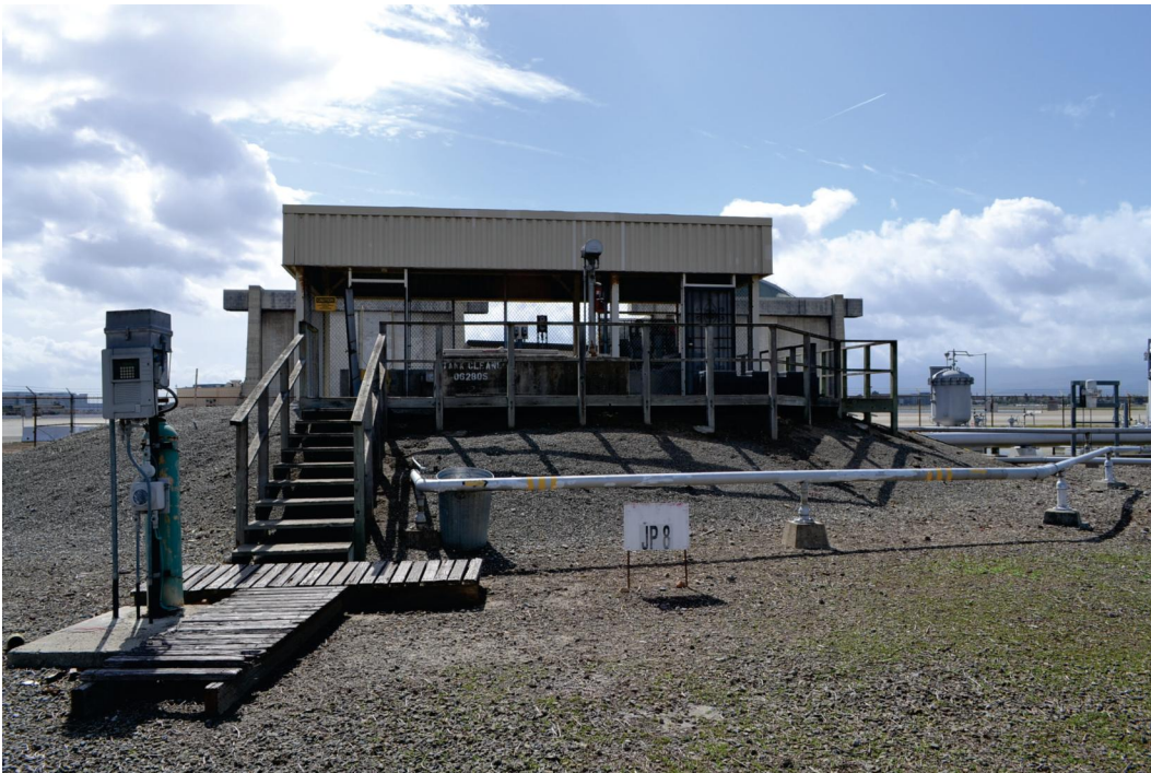
Plate 11. Building 953, view facing south (Hangars 2 and 3 in the background)
