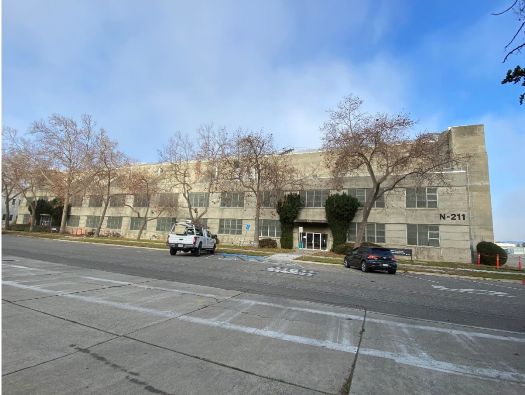
Photograph 3. South side of Building N-211 (offices), view facing north
