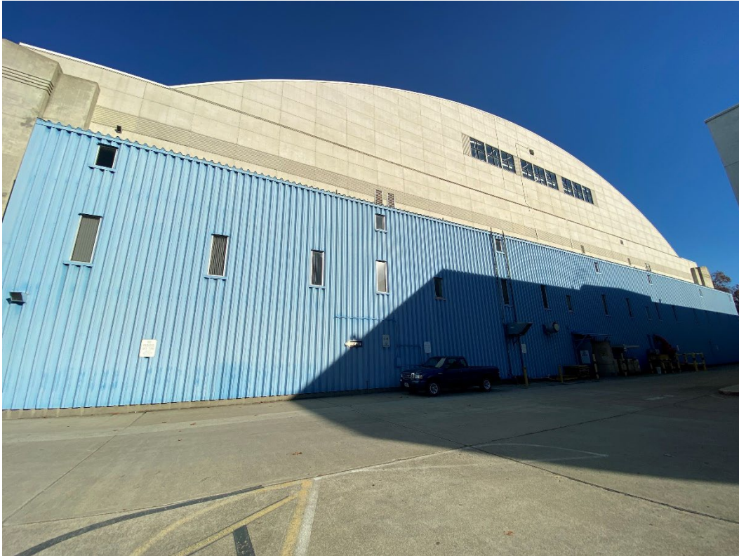
Photograph 2. West side of main hangar alteration, view facing east
