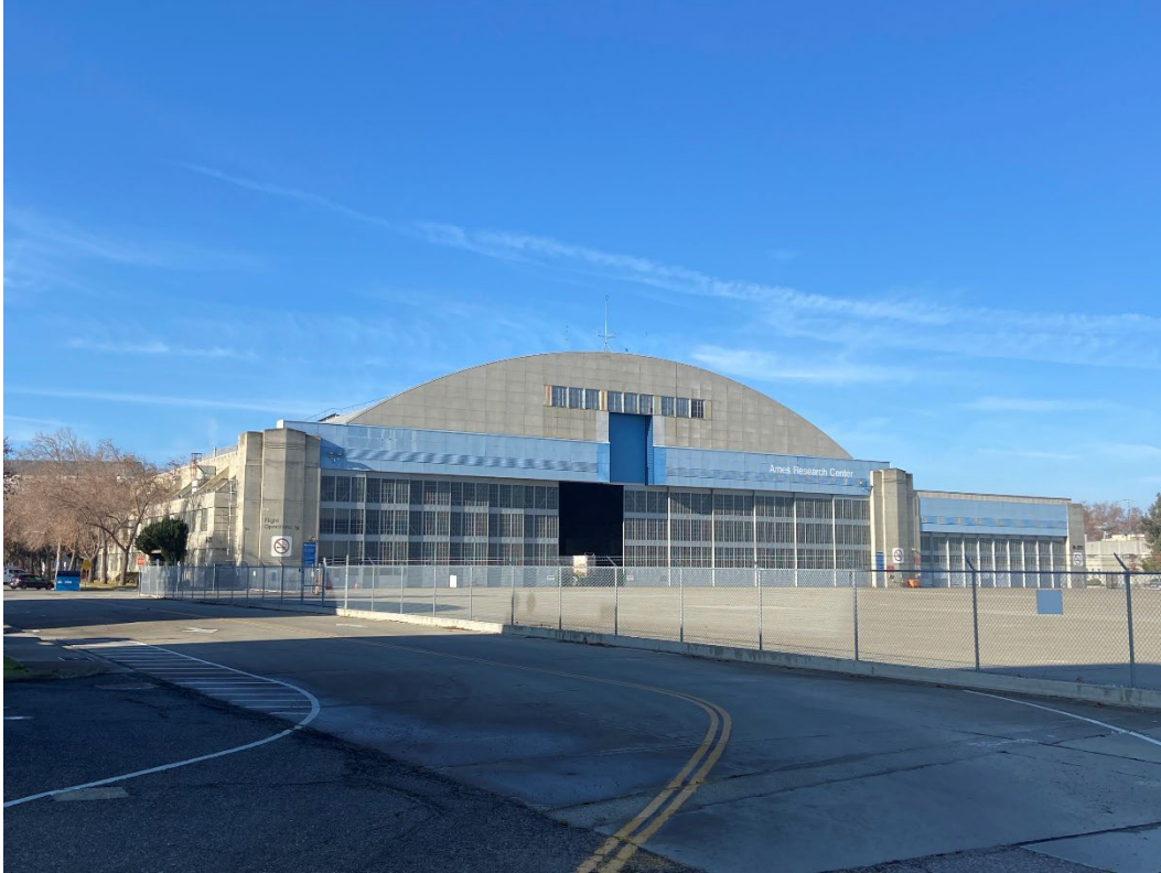
Photograph 1. East side of Building N-211 at the airfield, view facing west
