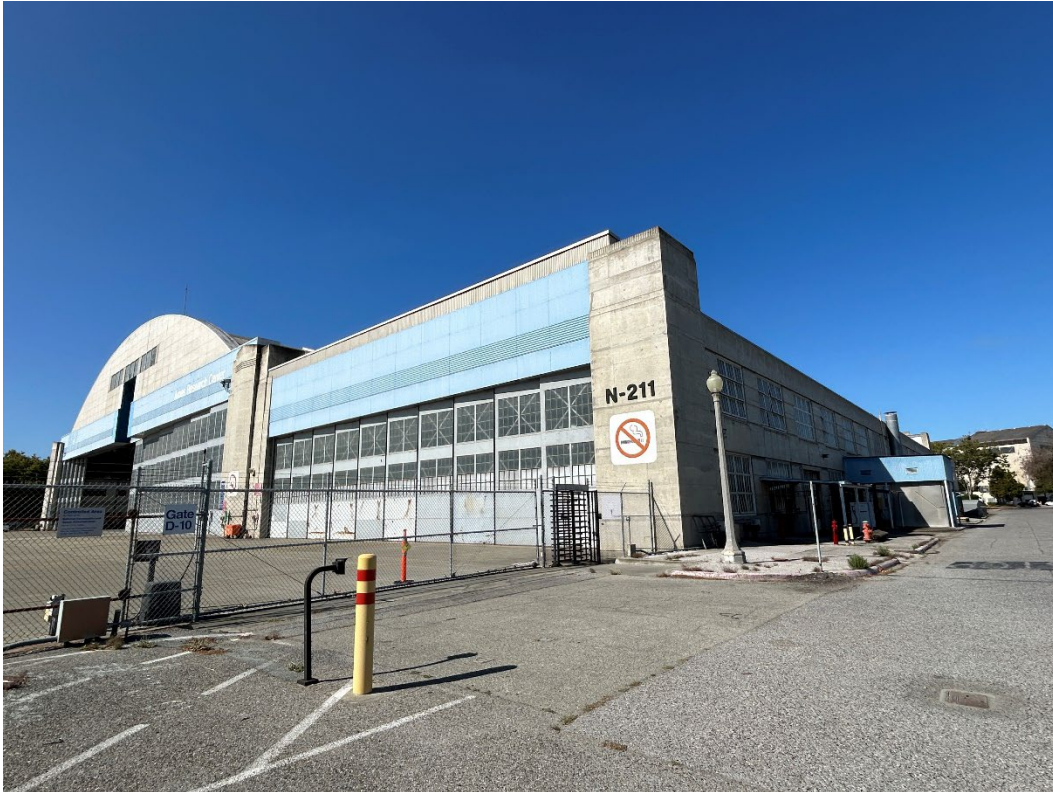
Photograph 4. East side of north hangar, view facing southwest
