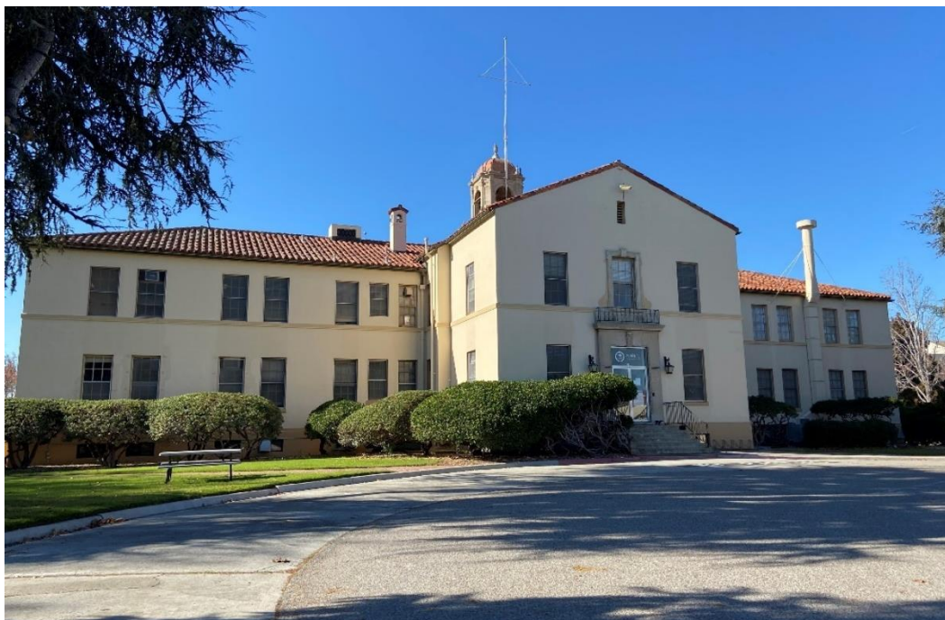
Photograph 2. Building 17, east (rear) elevation, view facing northwest
