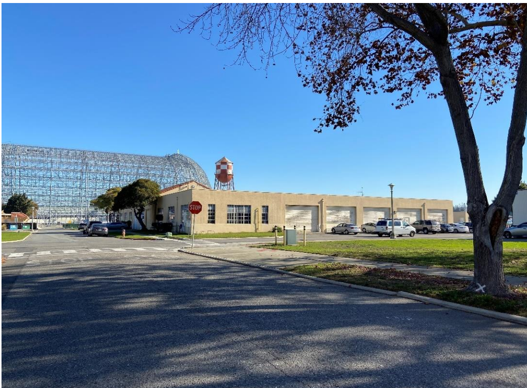
Photograph 7. Intersection of S. Akron Road and McCord Avenue, view facing southeast; Building T-36A at far right
