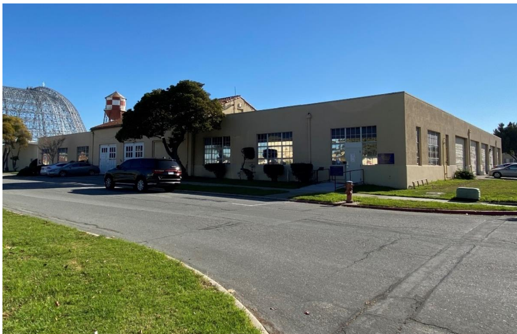
Photograph 1. Building 15, north and west elevations, view facing southeast
