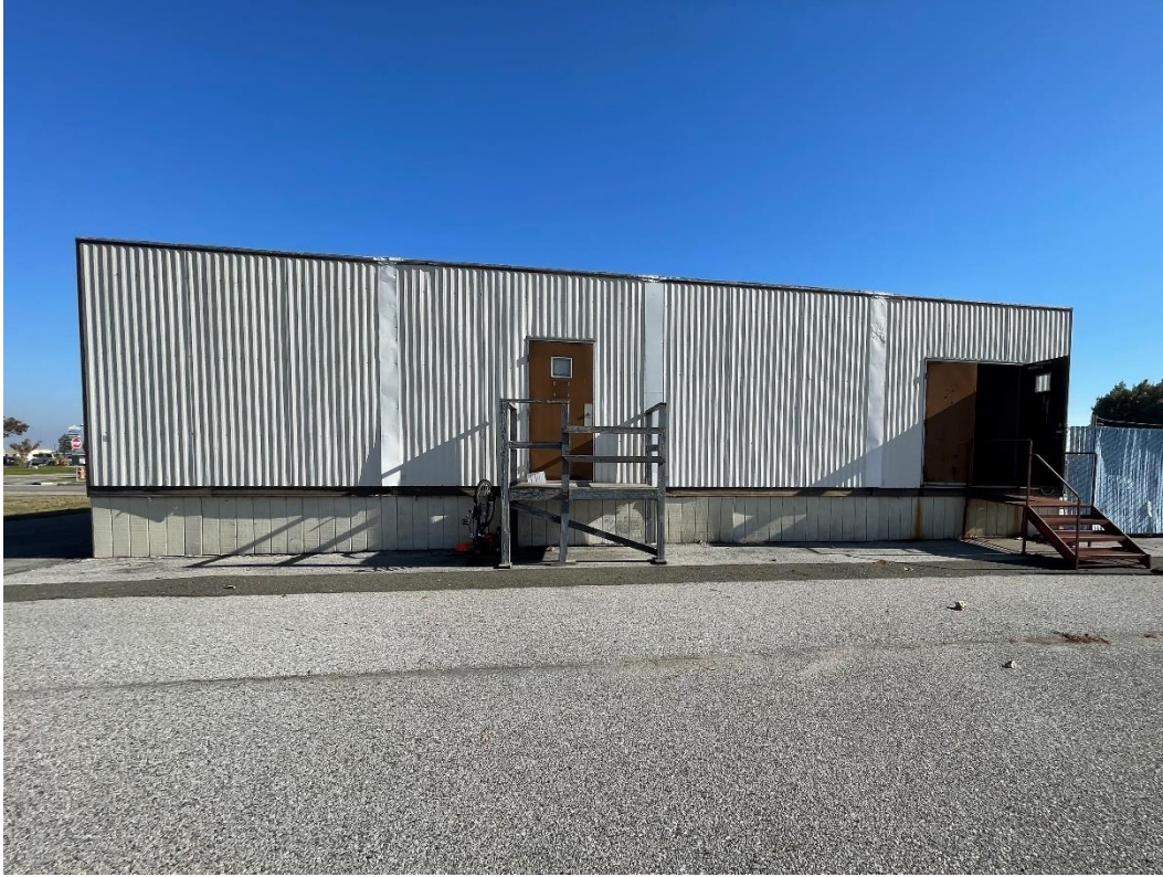
Photograph 3. Building T-36A, view facing northeast
