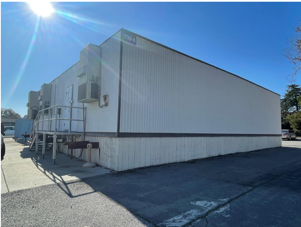
Photograph 6. Building T-36A, view facing south
