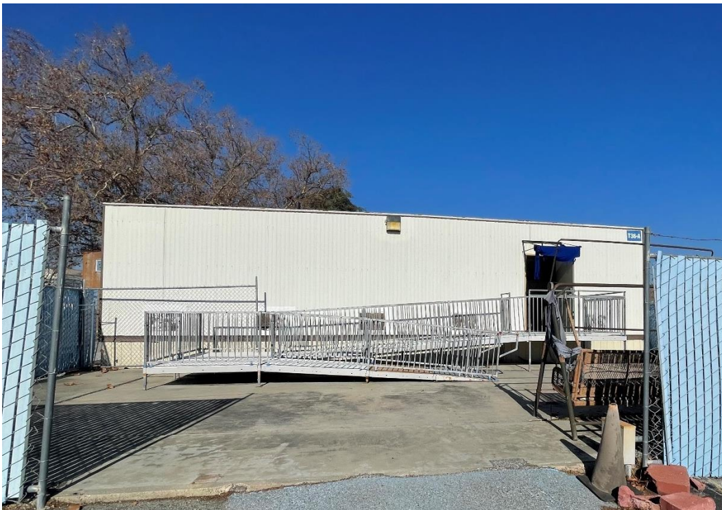
Photograph 4. Building T-36A, view facing northwest
