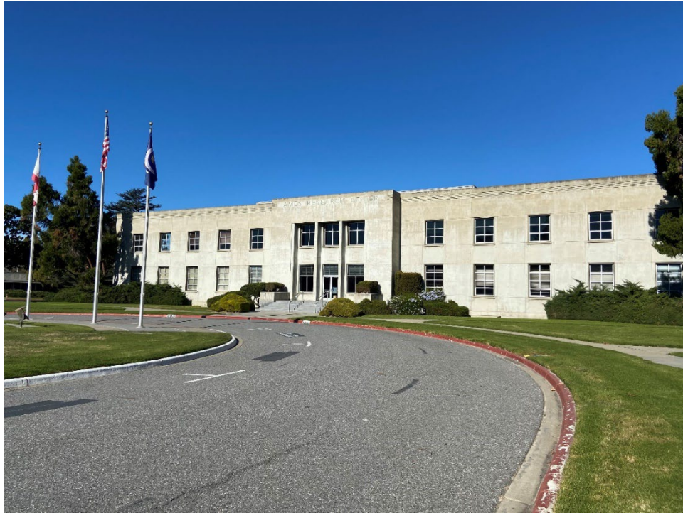
Photograph 1. Building N200 façade, view facing northeast
