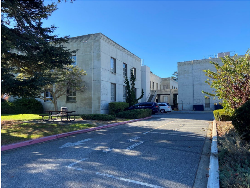
Photograph 2. Building N200 (rear) on left, exterior elevator shaft and staircase at center, and Building N201 at right, view facing southwest
