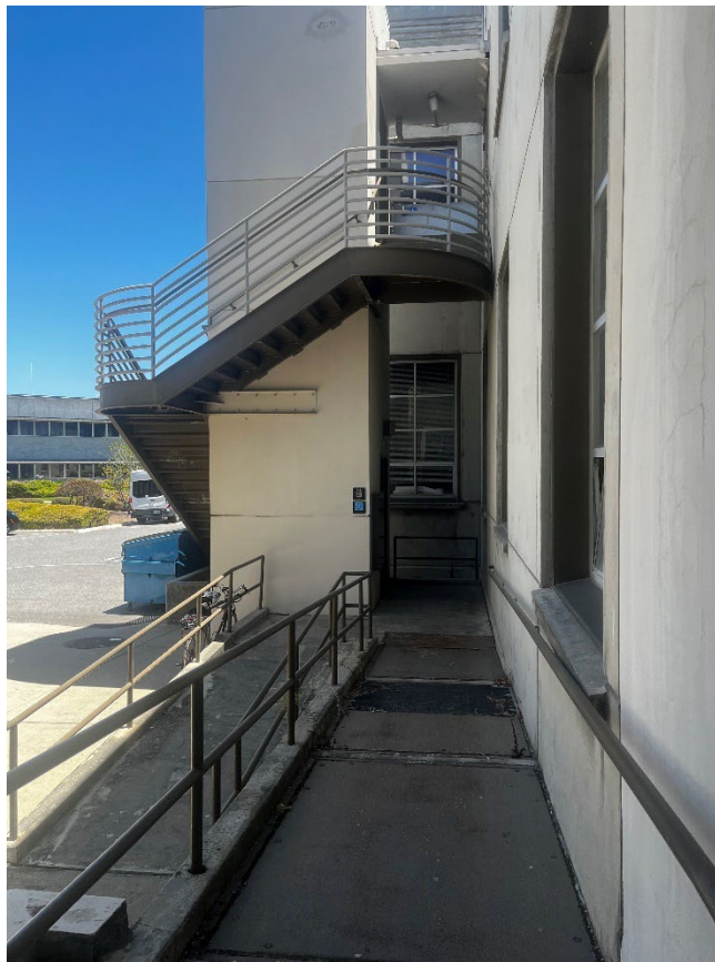
Photograph 3. Building N200 (rear), exterior elevator shaft and staircase, view facing southeast
