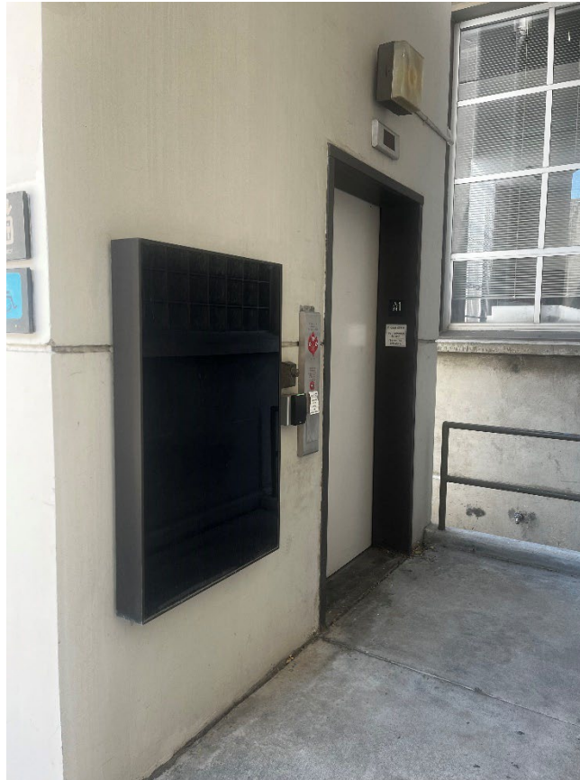
Photograph 4. Exterior elevator door and equipment on first floor, view facing northeast
