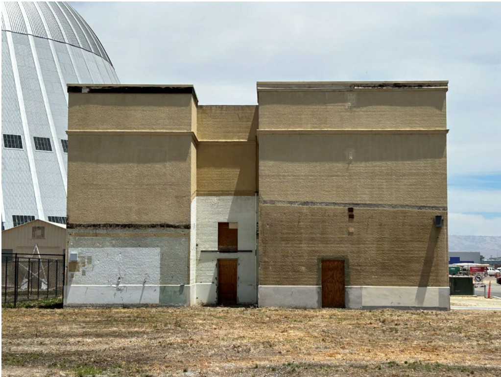
Photograph 4. Building 6, view facing northeast
