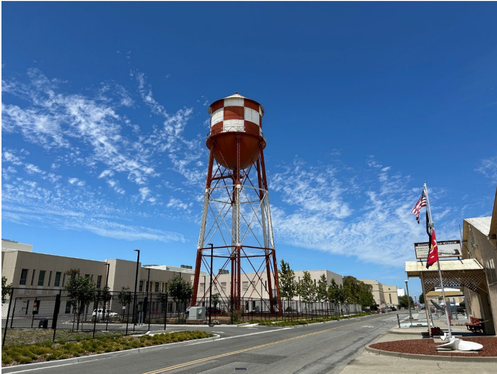
Photograph 1. Building 5 (Water Tower), view facing west
