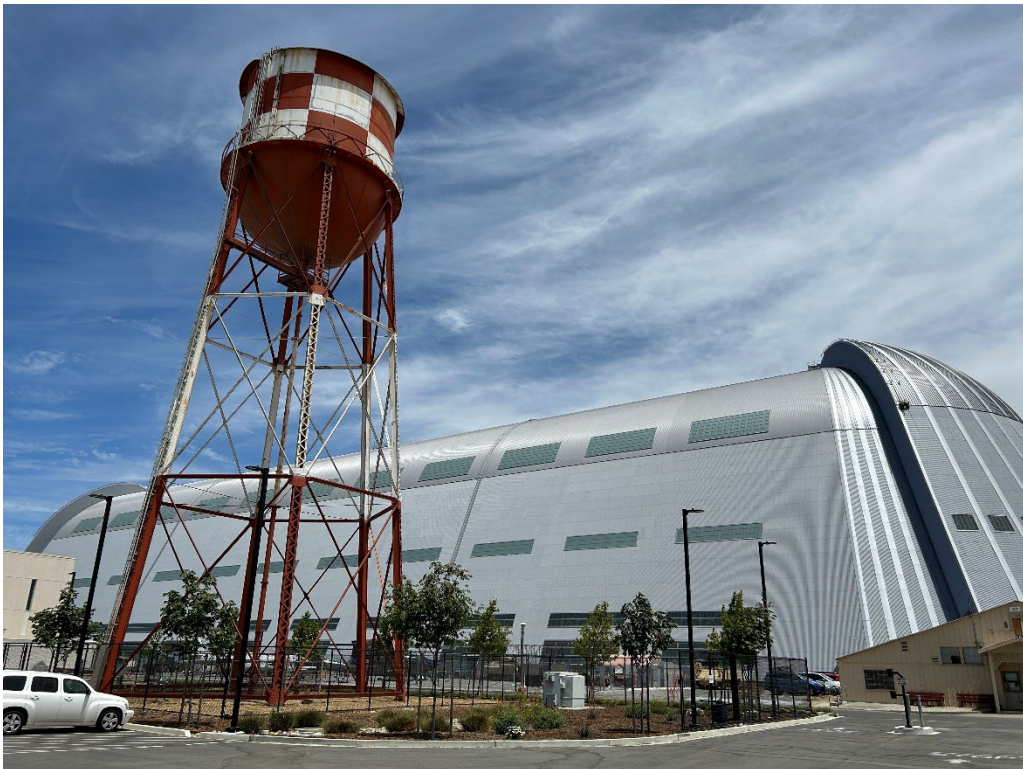
Photograph 2. Building 5 with Hangar One in background, view facing north
