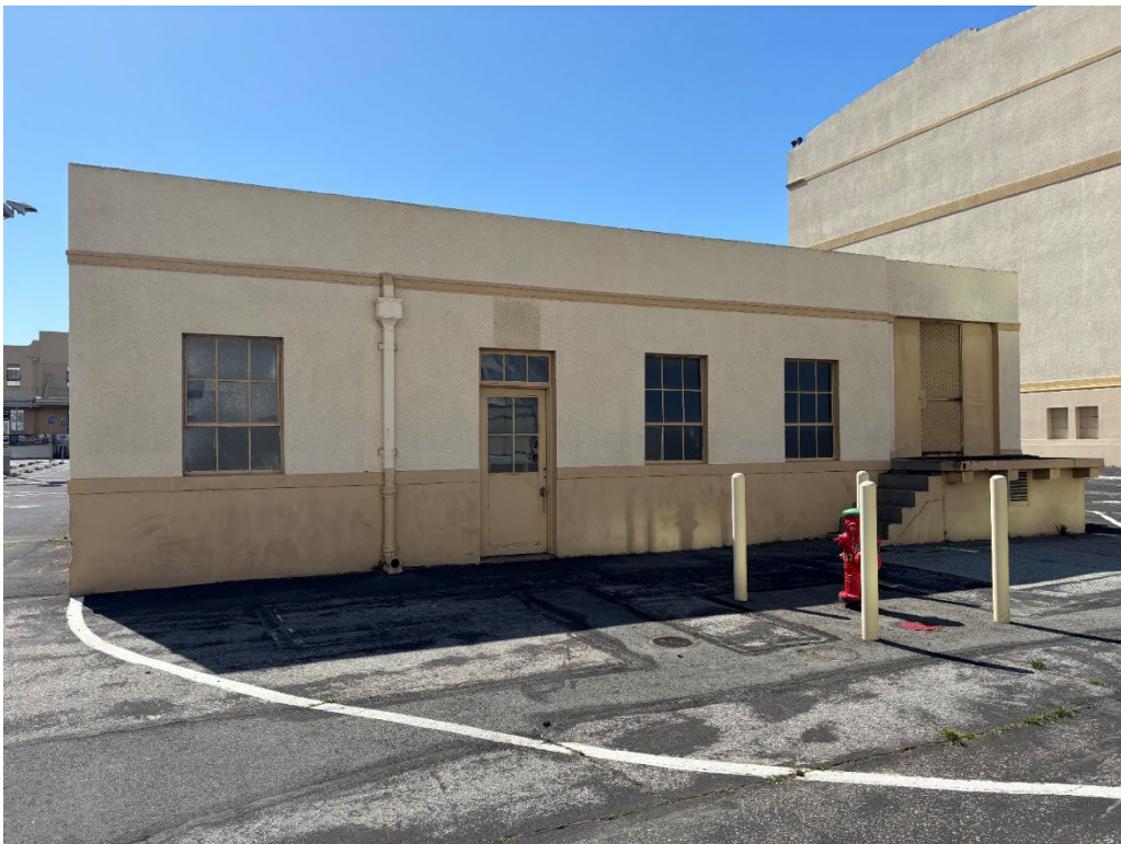
Photograph 6. Building 29, view facing southwest
