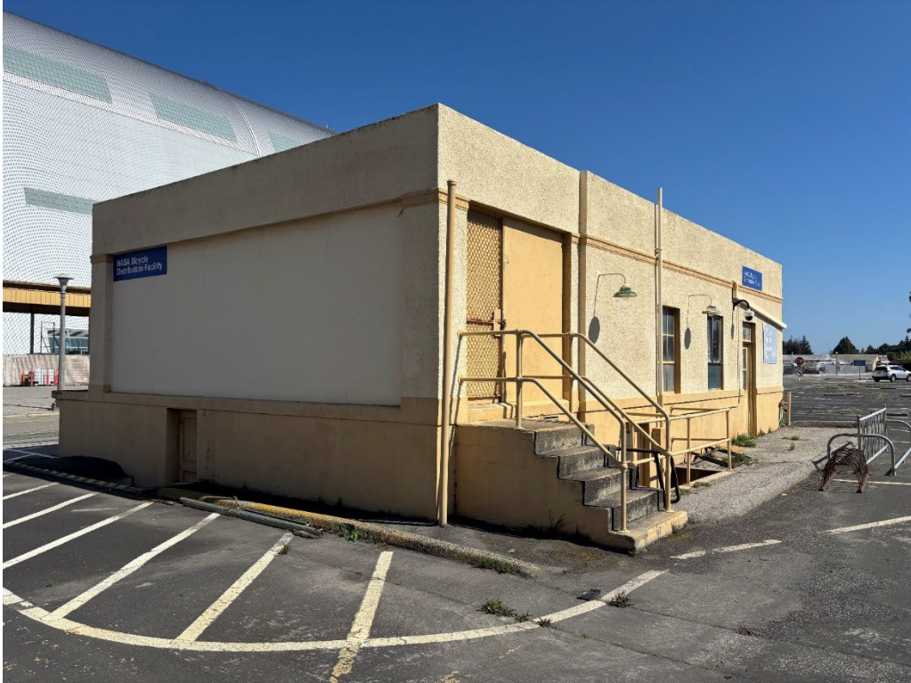
Photograph 5. Building 29, view facing east
