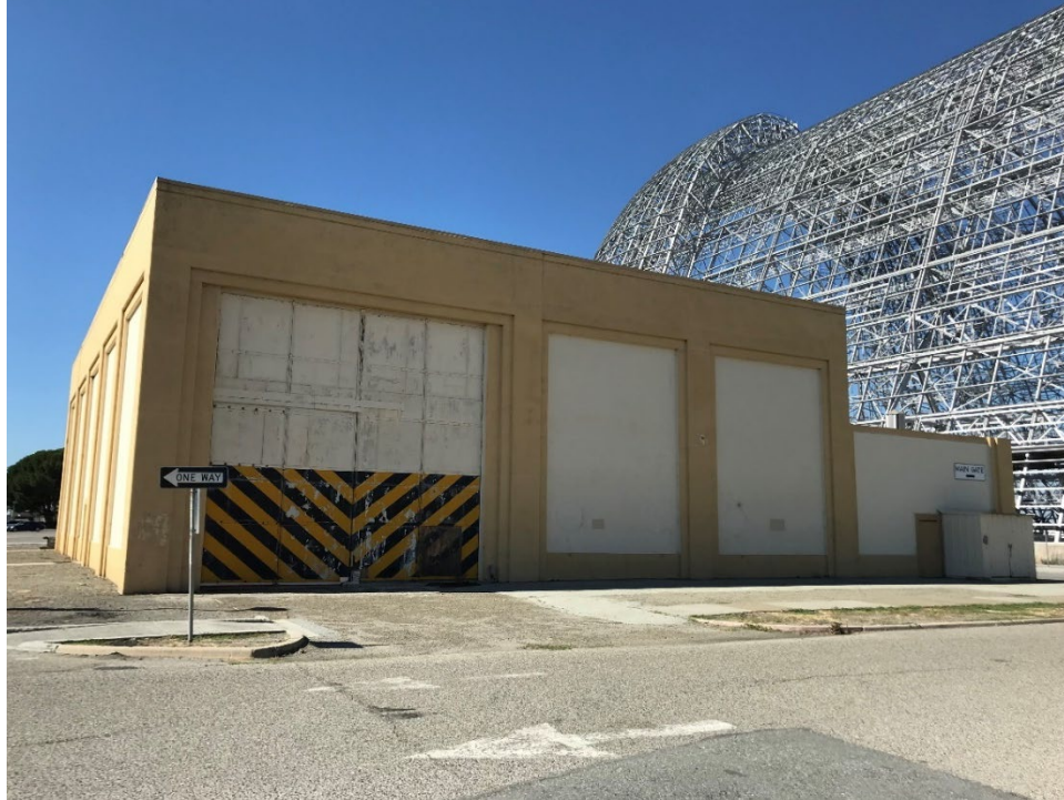
Photograph 1. Building 45, west and south sides, with Hangar 1 in background, view facing northeast.
