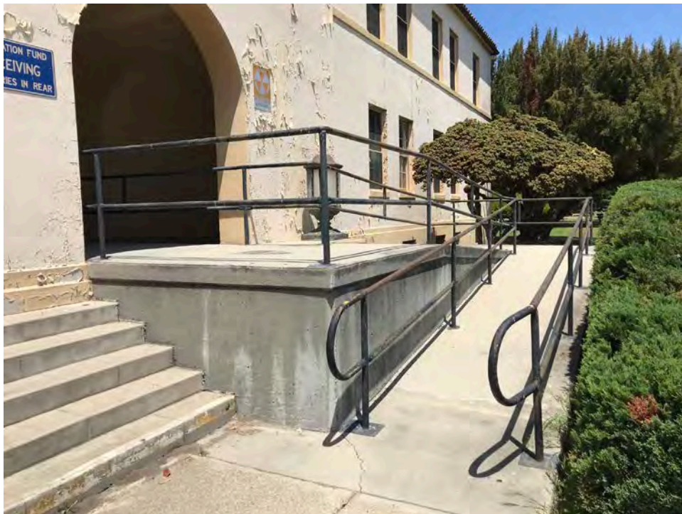
Plate 10. Building 25, concrete ramp addition at main entrance, view facing northeast.
