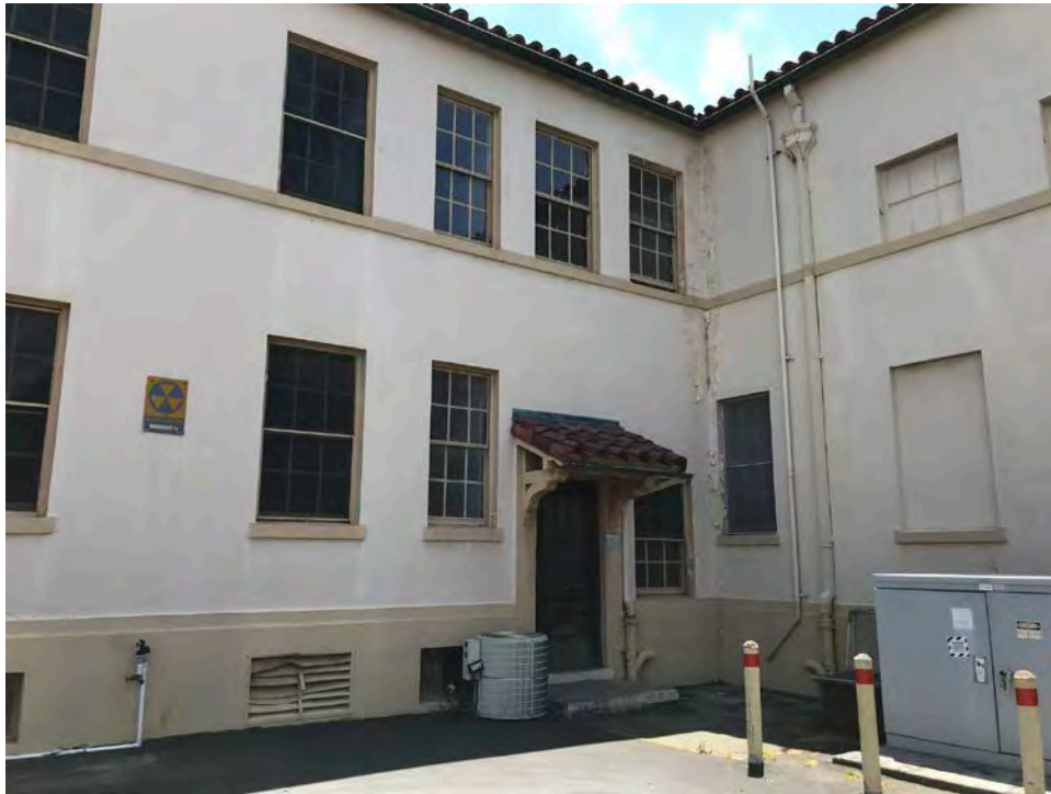
Plate 9. Building 25, typical fenestration at rear, view facing southwest.
