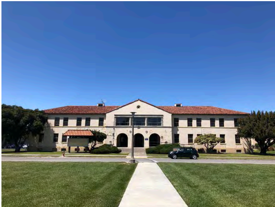
Plate 6. Building 25, view facing northwest.
