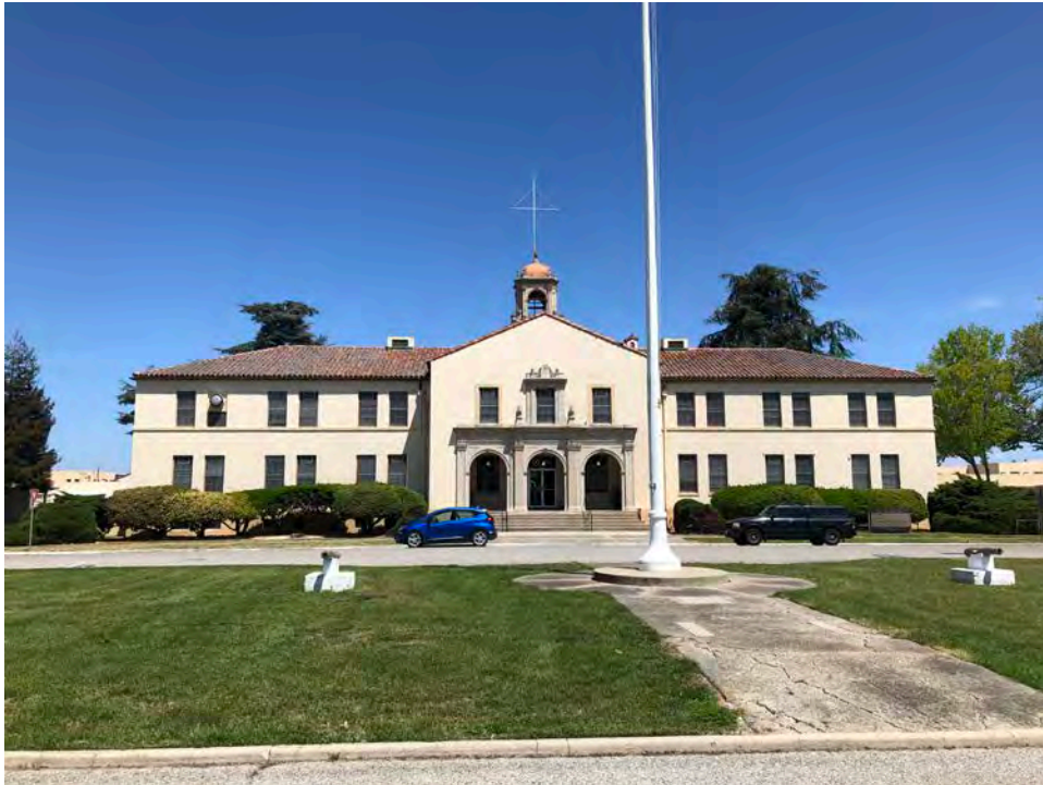
Plate 2. Building 17, view facing northeast.
