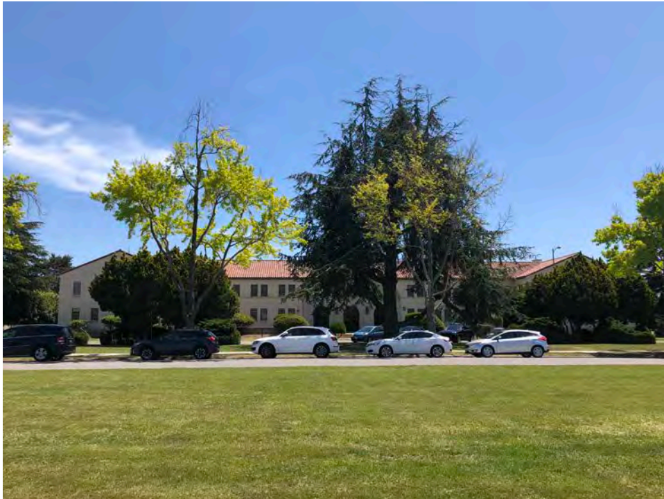
Plate 4. Building 20, view facing southeast.
