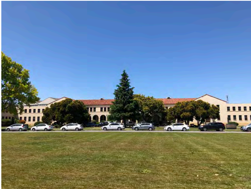
Plate 3. Building 19, view facing northwest.
