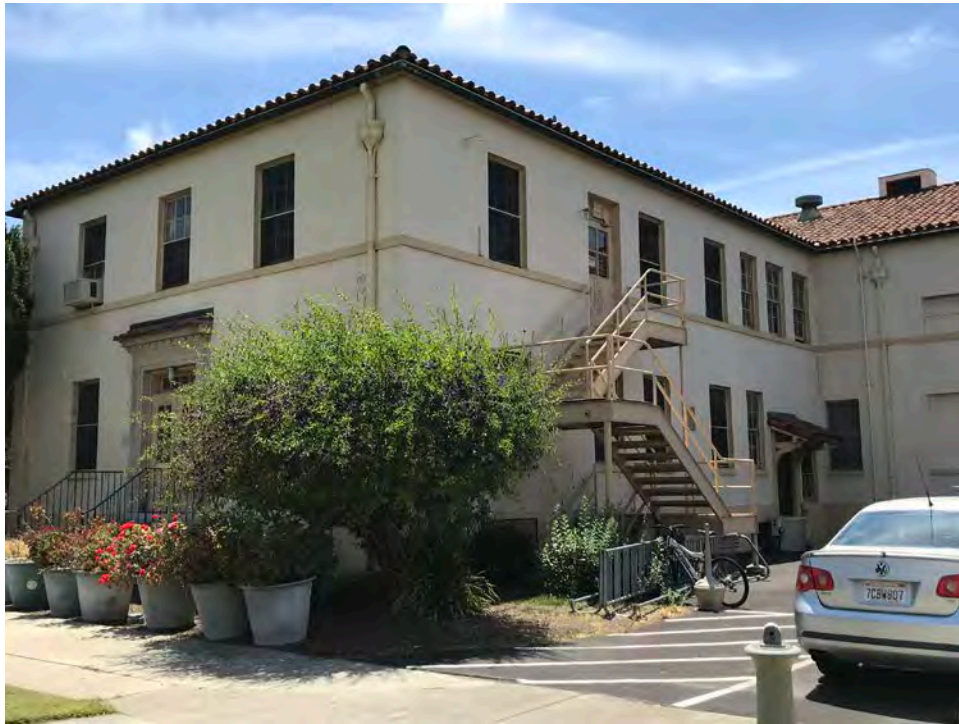
Plate 11. Building 25, metal stair addition at rear, view facing southwest.
