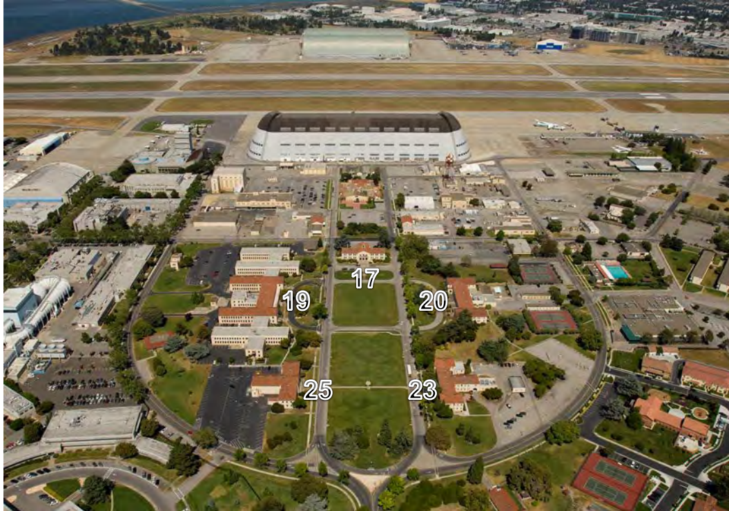
Plate 1. Shenandoah Plaza overview (center), showing Buildings 17, 19, 20, 23 and 25.
