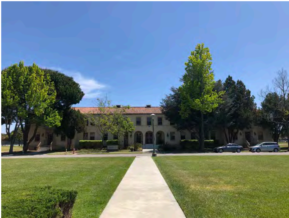
Plate 5. Building 23, view facing southeast.
