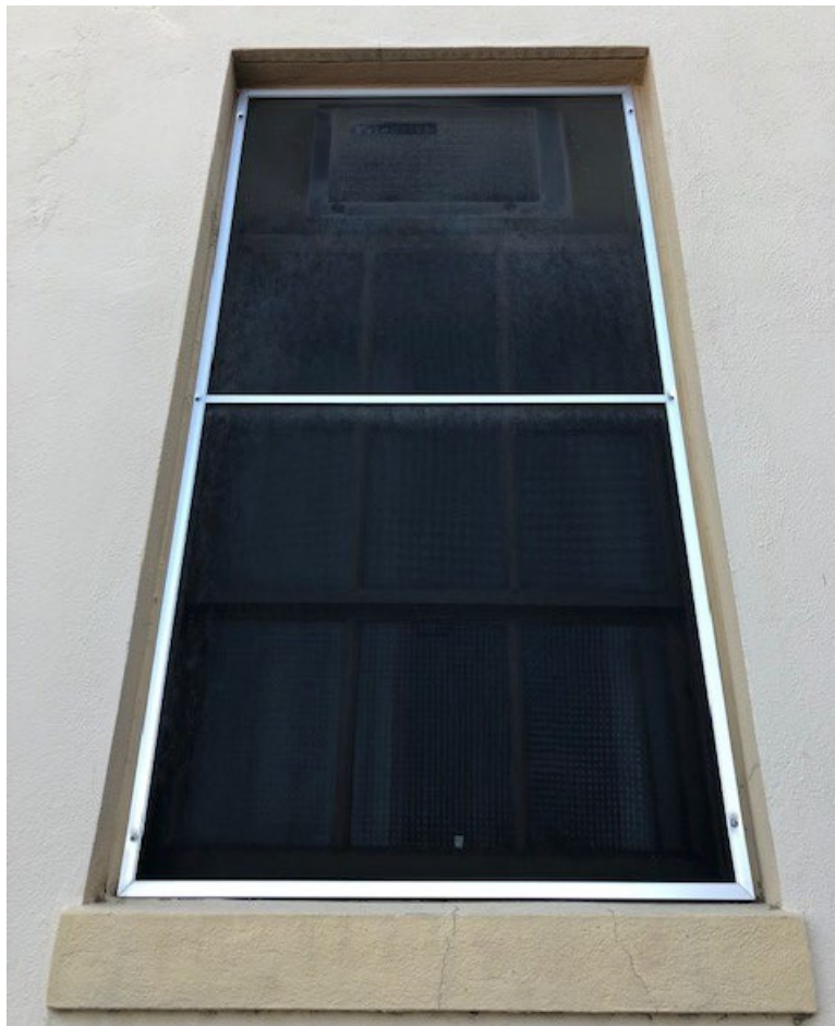
Photograph 8. Detail of typical six-over-six metal sash window with screen.
