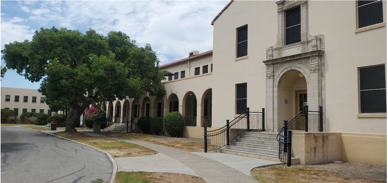
Photograph 3. Building 19 façade (south elevation) showing arcaded loggia in the story between the two shallow gable roof projections. Eastern projection in foreground on right and western projection obscured by tree in background at center-left, view facing northwest.
