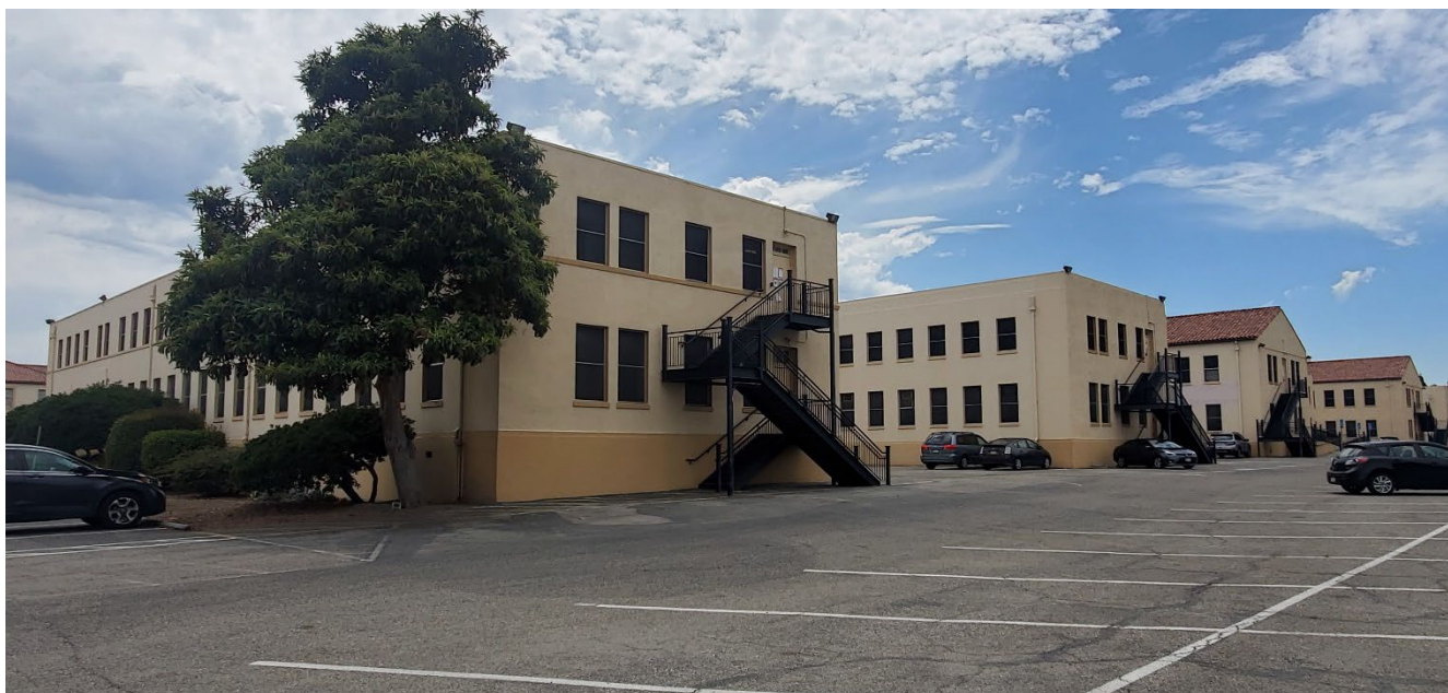
Photograph 6. Building 19 rear, north elevation, 1952-constructed eastern wing additions in foreground, view facing west. The red tile roof sections are part of the original 1933 building.
