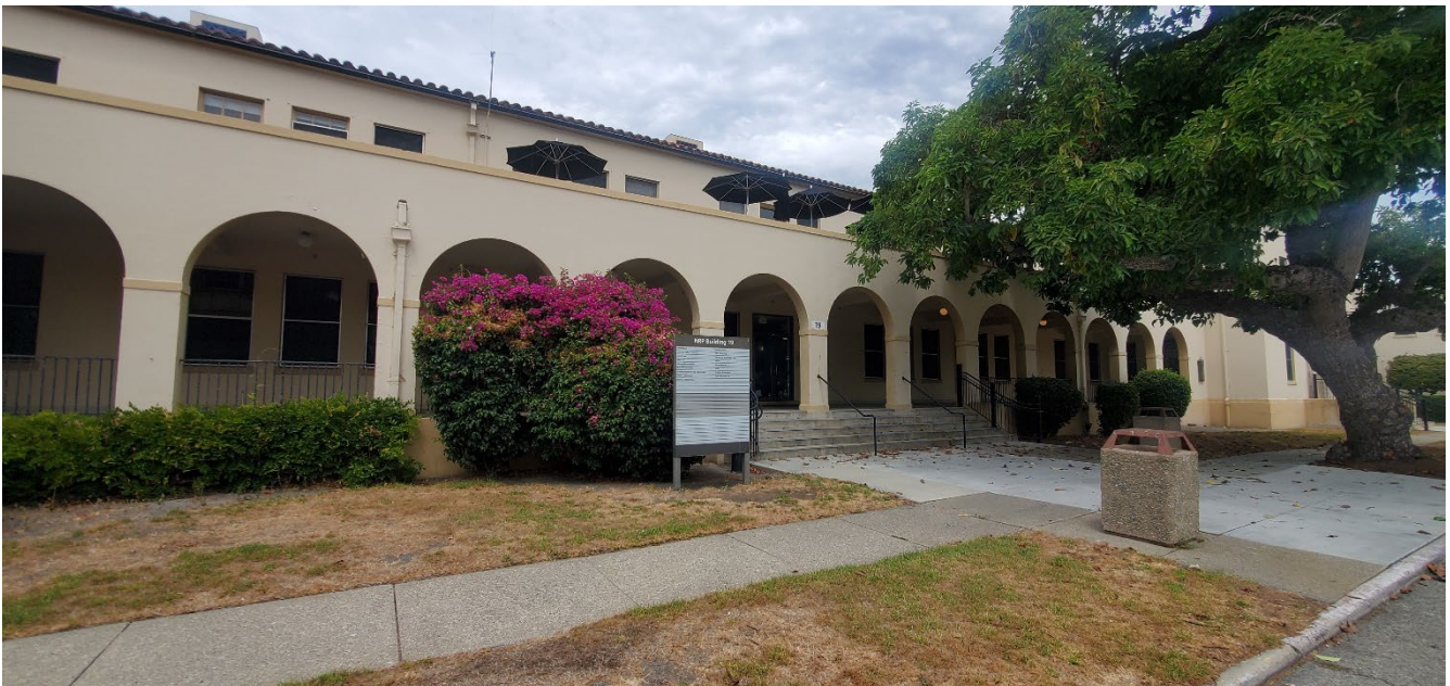
Photograph 4. Building 19 façade (south elevation) showing arcaded loggia in the first story, with eastern projection on far right, view facing northeast.
