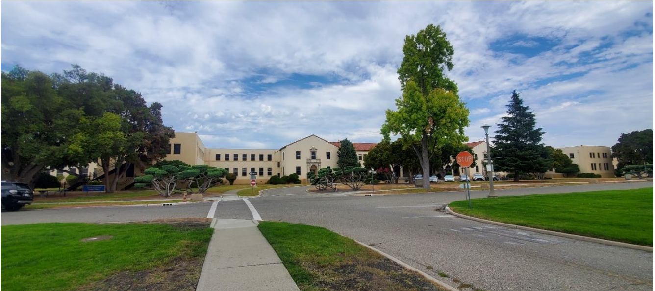
Photograph 1. Building 19 façade (south elevation), view facing north. The red tile roof section is the original 1933-constructed building and Conference Room 1218 is located behind the stop sign.
