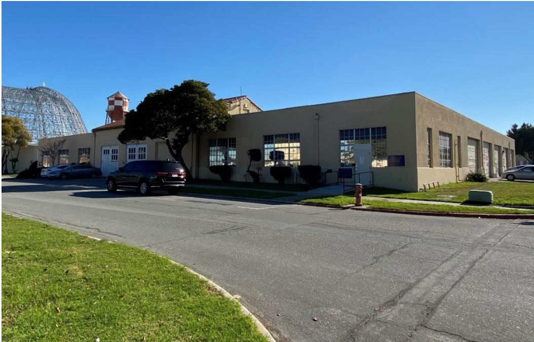
Photograph 3. Building 15, north and west elevations, view facing southeast
