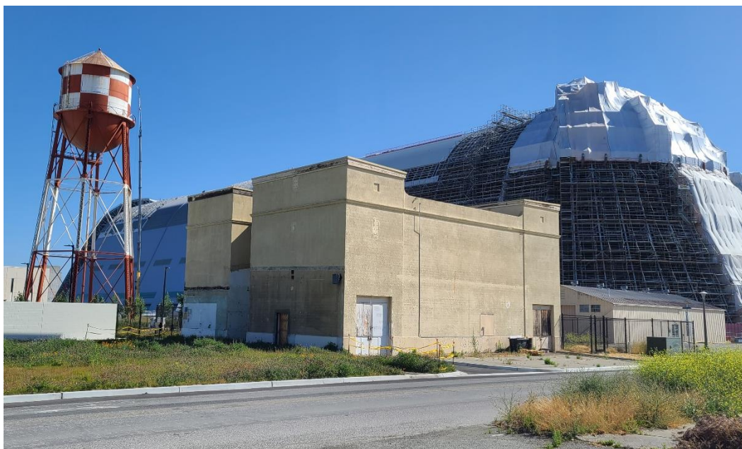
Photograph 1. Building 6, west and south elevations, with Hangar 1 in background, view facing northeast. The west elevation of Building 6 faces the project site
