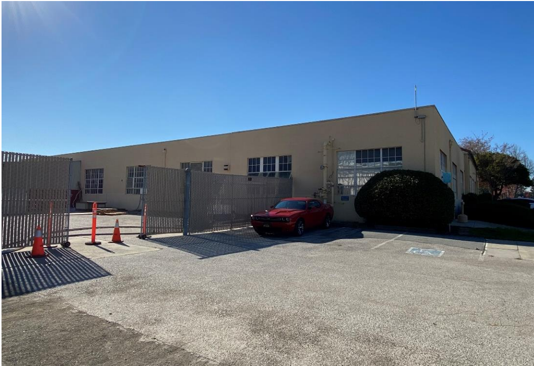
Photograph 7. Building 15, east elevation with existing gate and fencing that will be replaced by the current project, view facing southwest
