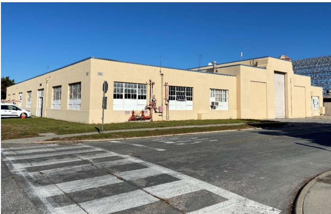
Photograph 4. Building 16, south and west elevations, view facing northeast
