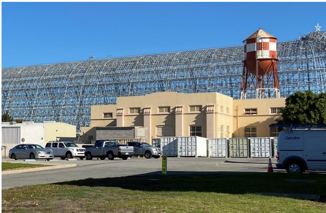
Photograph 2. Building 10 in foreground, west elevation facing the project site, view facing northeast
