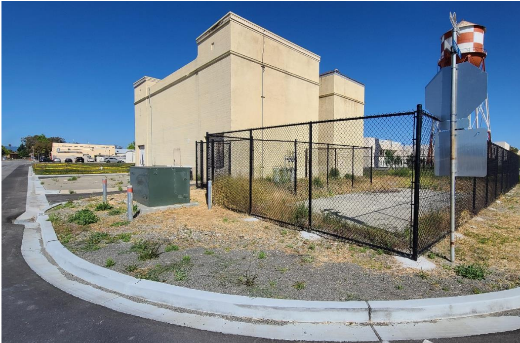
Photograph 9. Building 6 in foreground, project site with east elevation of Building 16 on far left and portion of Building 510 at center, to be enclosed with new fencing, view facing northwest
