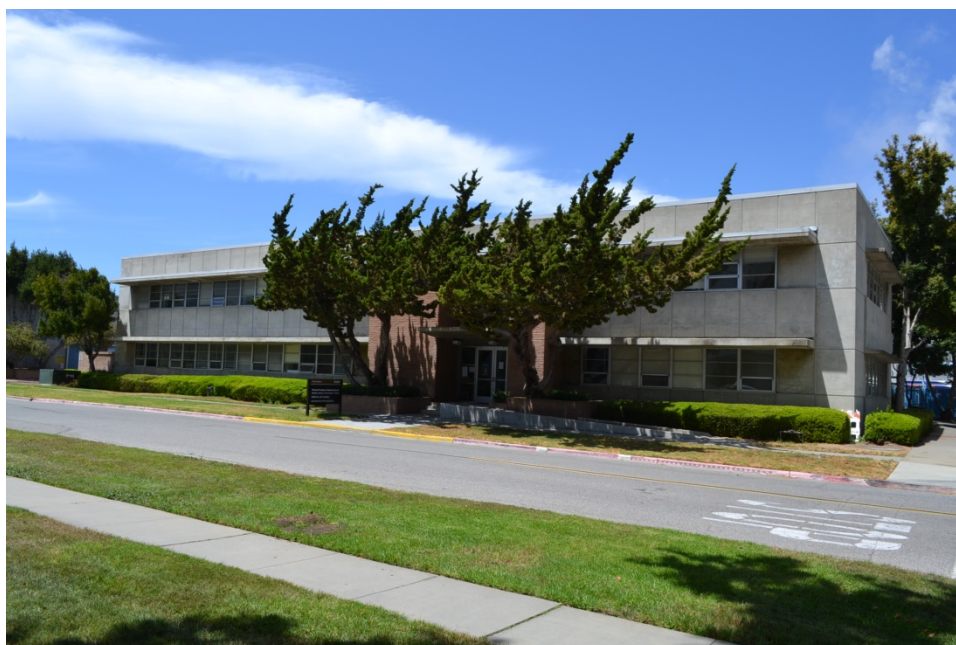
Plate 2. Building N234, view facing northwest.
