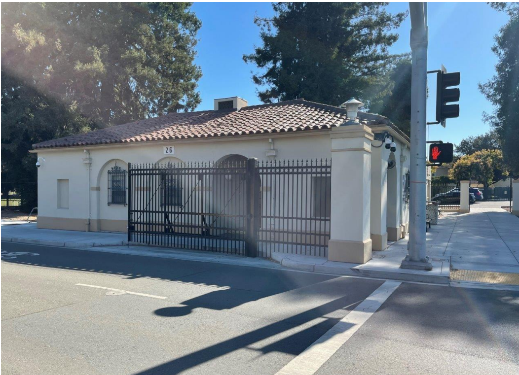
Plate 3: North side of Building 26 and gate, view facing southeast, November 7, 2024.
