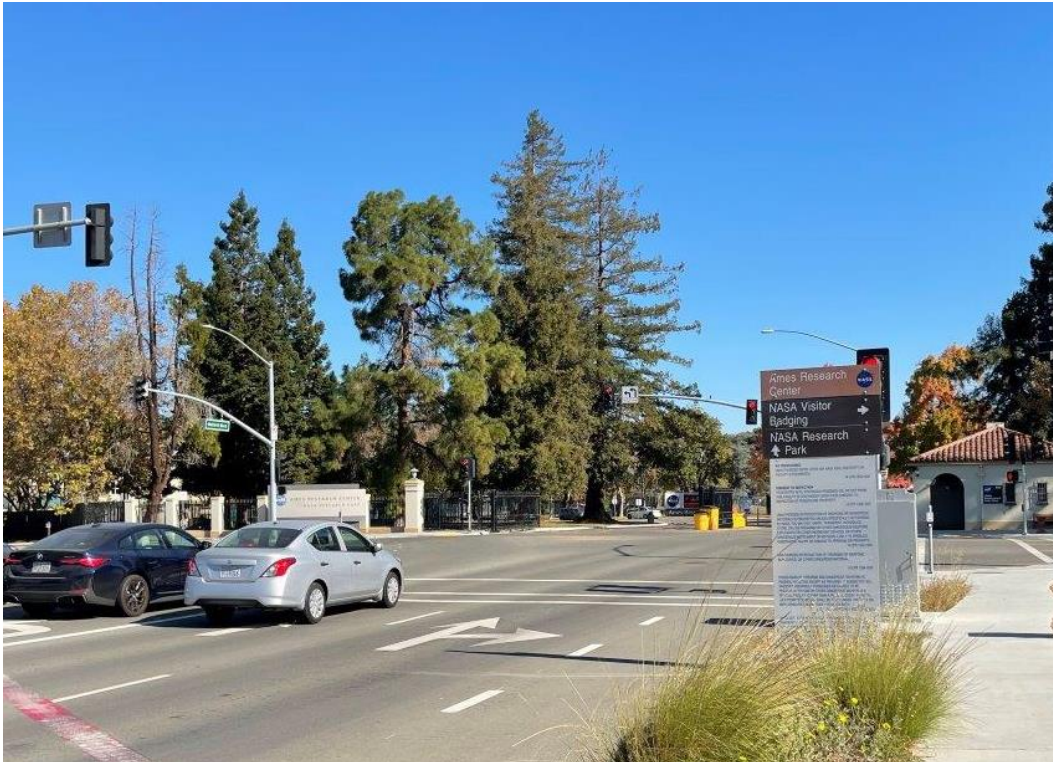
Plate 4: Overview of modified gates and gate posts, view facing northeast, November 7, 2024. Compare to Plate 5 below.
