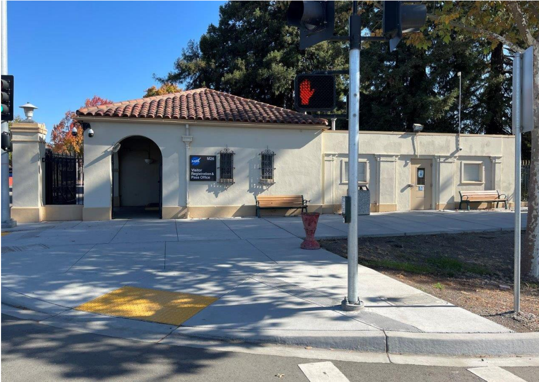
Plate 2: West side of Building 26, view facing east, November 7, 2024.
