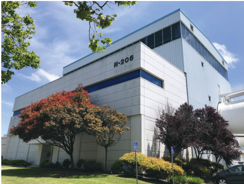
Plate 2: Building N206, the 12-foot Pressure Wind Tunnel, view facing southeast.
