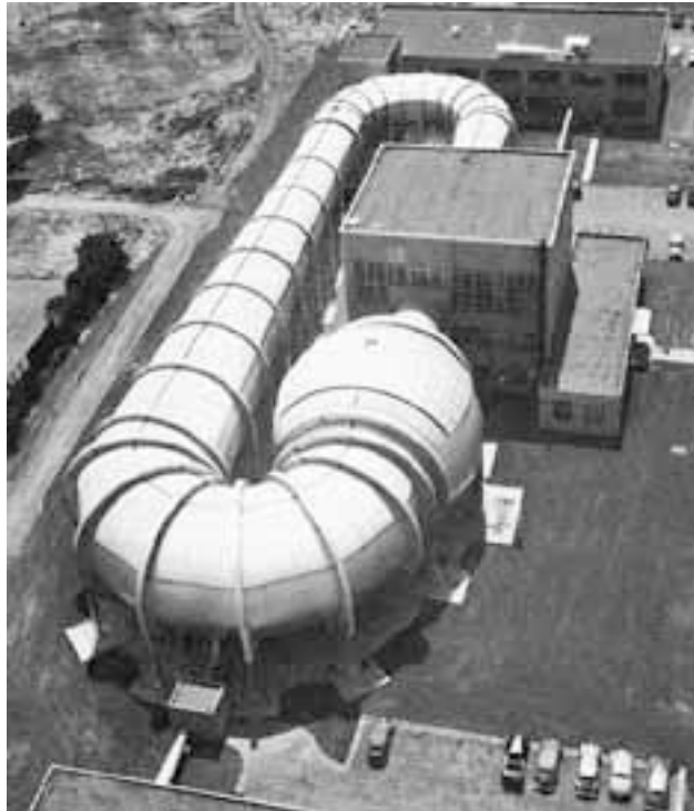
Plate 1. The original 12-foot Low Turbulence Wind Tunnel, 1946. (Source: Hartman 1970)
