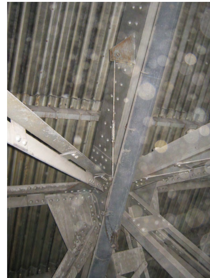
Figure 3-26: Typical Pipe Support at Hangar Wall
