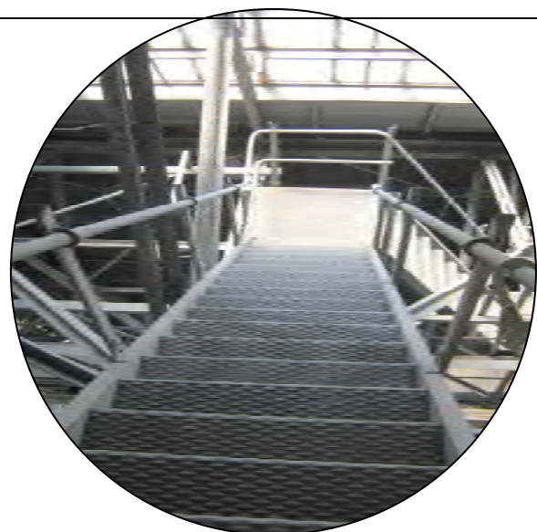
Figure 3-2: Stairs Between Catwalks
