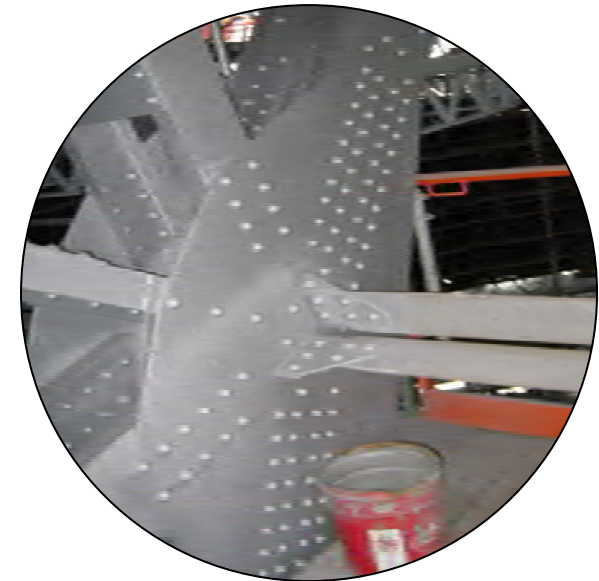
Figure 3-11: Bottom Chord Connection
