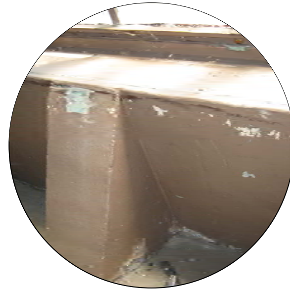
Figure 3-16: Concrete Wall at Hangar Perimeter, From Inside
