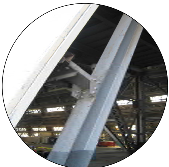
Figure 3-4: Wind Girt @ 7'-6" O.C.
