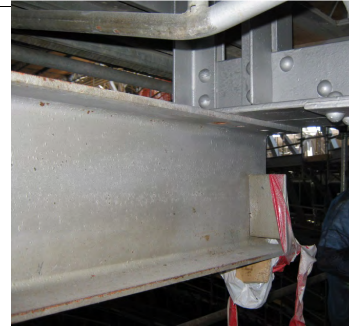
Figure 3-25: Crane Beam End Connection
