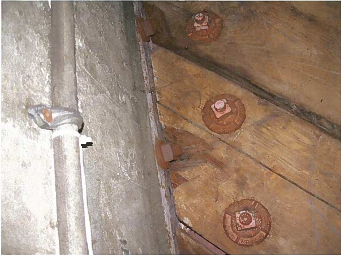
Figure 10. Truss to concrete tower wall connection.
