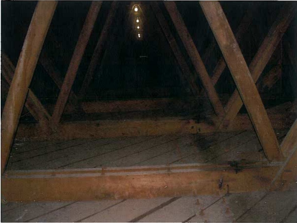
Figure 5. Inside of main truss showing transverse support trusses.
