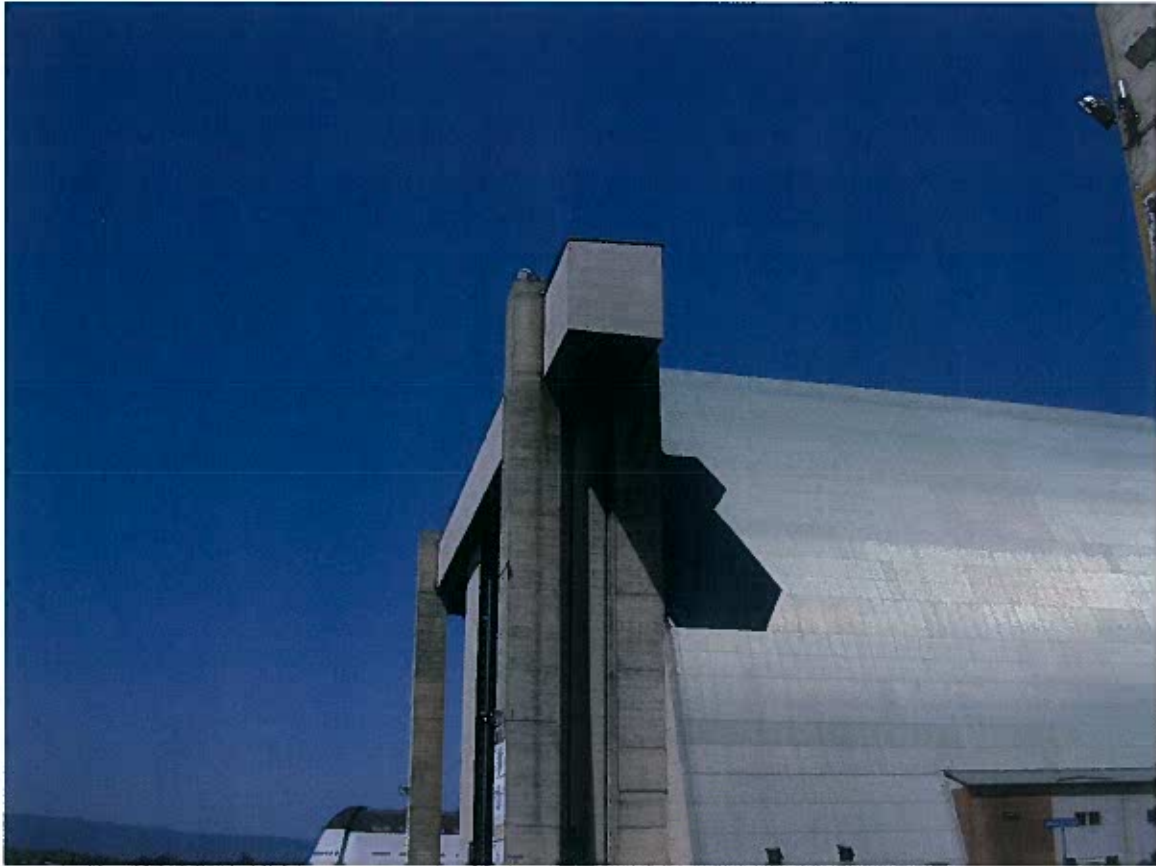
Figure 1. Existing truss and support towers.
