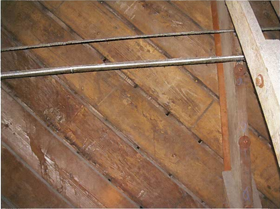
Figure 4. Photograph showing the overlapping 3x truss members.
