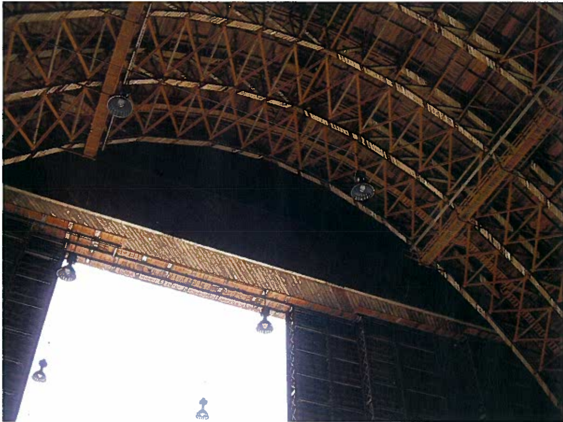
Figure 3. Truss viewed from inside hangar.
