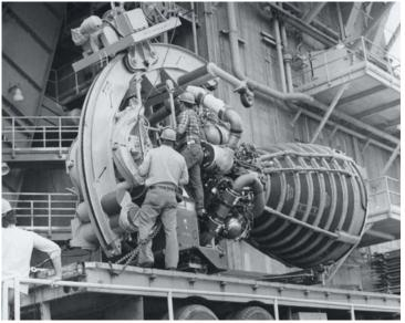
Photo 2.2. SSME hoisted into the A-2 test stand at Stennis Space Center (then, NSTL) before undergoing test firing, January 1, 1979. (Source: NASA-HQ-GRIN; GPN-2000-000546)
