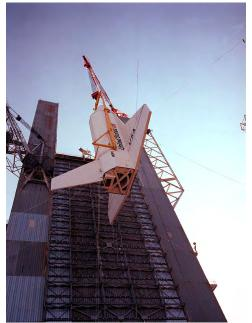
Photo 3.3. Pathfinder Simulator is hoisted into MSFC Dynamic Test Stand, 1977. (Source: NASA MSFC, NIX No.: MSFC-7885689)
