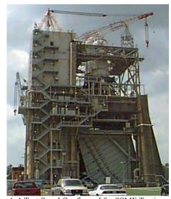
A-1 Test Stand Configured for SSME Testing. (Source: Stennis Space Center 2007:32)
